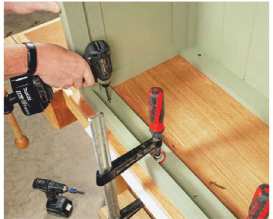
When the finish on the top panel cures, install it on the cabinet by driving washerhead or pocket screws through the stretchers into it. Allow for a 1" overhang on the front edge and ends.
