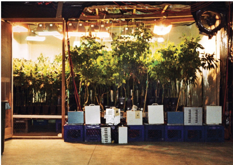
All electrical wiring and components must always be kept off the floor and away from contact with water, for obvious reasons.
