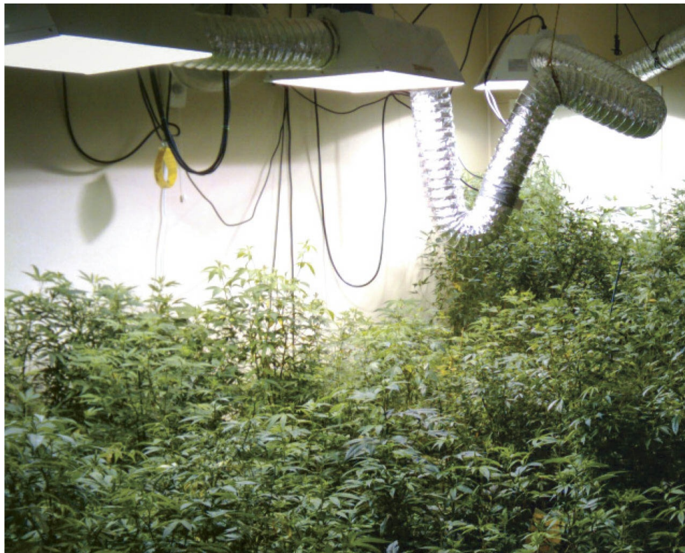
Air-cooled lighting setup in clone mother room. Photos: Cannanetics
