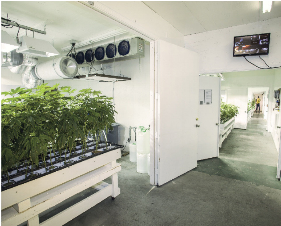
Chambered grow operation with ventilation, air filtration, and security systems visible.
