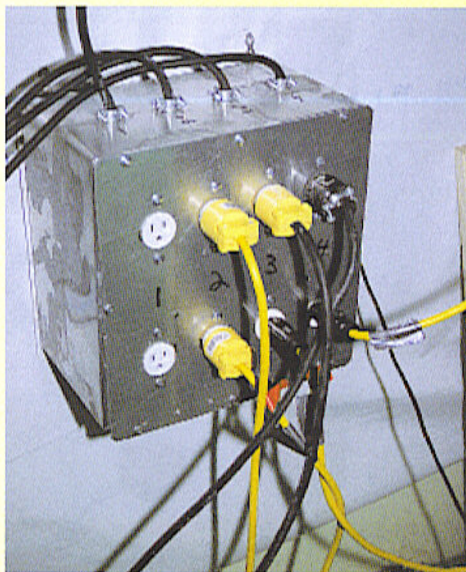
BC growers run flowering rooms 24 hours a day with half as many ballasts. This box is made for three transformers, capacitors, and starters to run six 1000-watt HP sodiums. Three lamps run for 12 hours; the other three lamps run for the next 12 hours.
