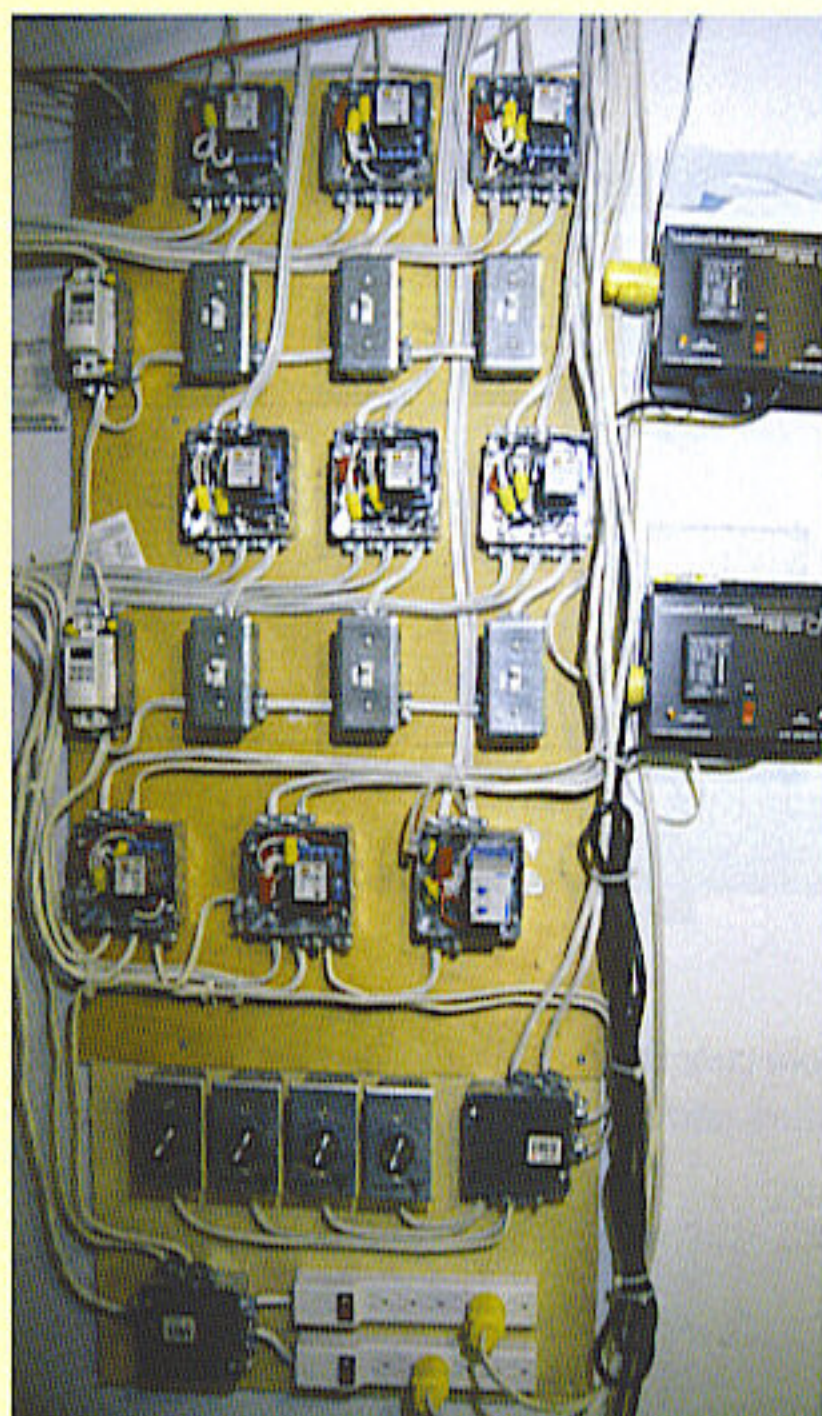
Fixing all wiring and electric devices to a control panel makes control and troubleshooting easy.
