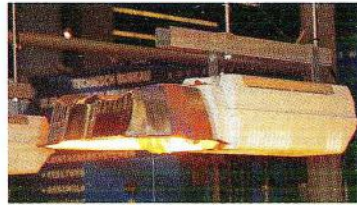
If ballast is attached to the fixture, hooks should be strong enough to support 30 pounds (14 kg) for each lamp.
