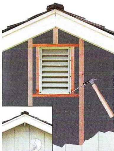
Install a vent in the attic
