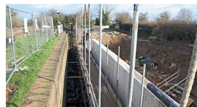
Hurleston lock wall being rebuilt in concrete
