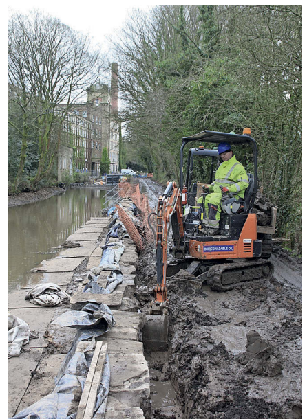
Backfilling the towpath wall with puddled clay
