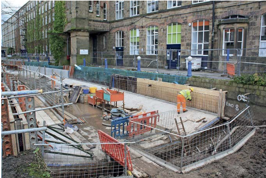
The new reinforced concrete canal channel taking shape in Bollington
