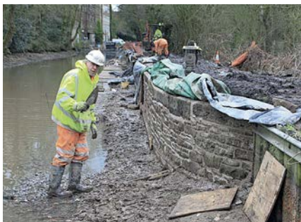
Pointing the rebuilt stone towpath wall
