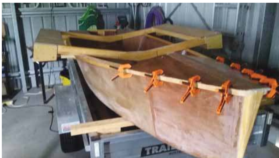
TOP: Starting Tryst construction.
