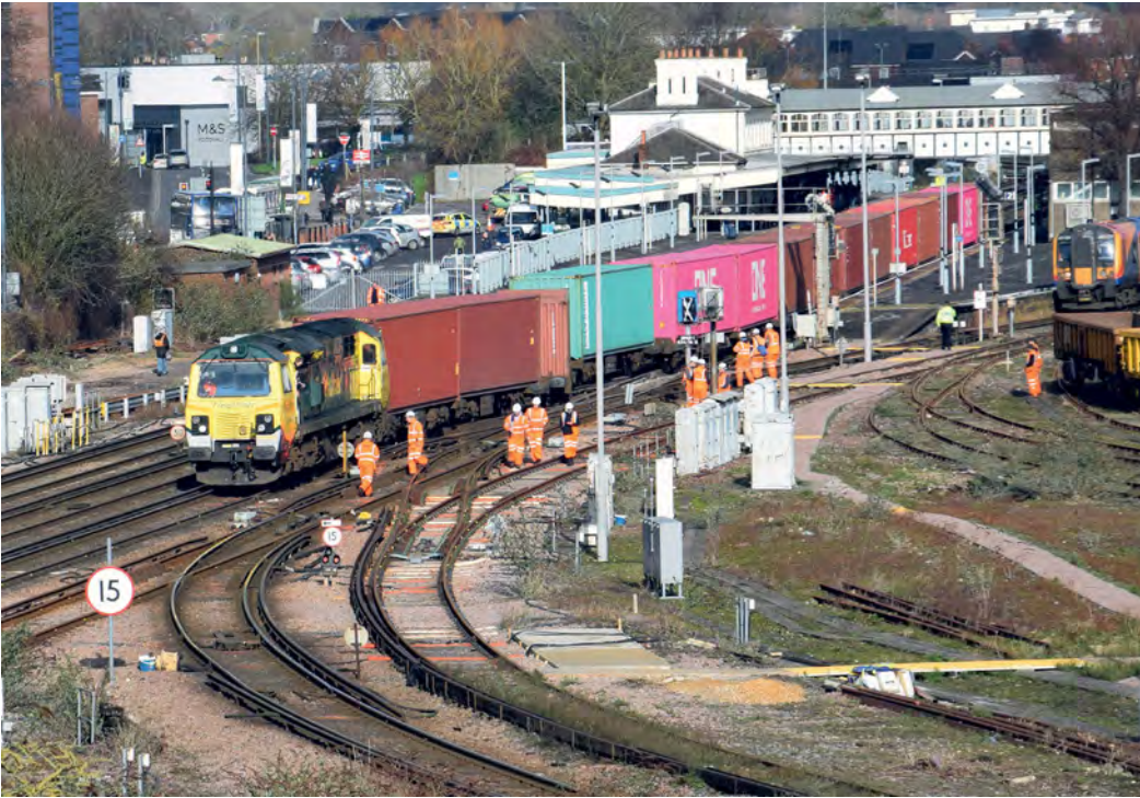
The Freightliner-operated 4005 Birch Coppice to Southampton intermodal working derailed at Eastleigh on January 28, causing considerable damage to the trackwork. SWR services were severely disrupted for six days while the six derailed loaded container flats were removed and temporary plain track was laid. Track spread has been identified as the cause. New points have to be produced and reinstalled, so disruption was expected to last into March. (Carl Watson)
