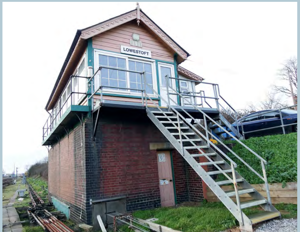
An external view of Lowestoft signal box on December 18, 2019. Note the extensive point rodding and signal wires exiting the base of the box.
