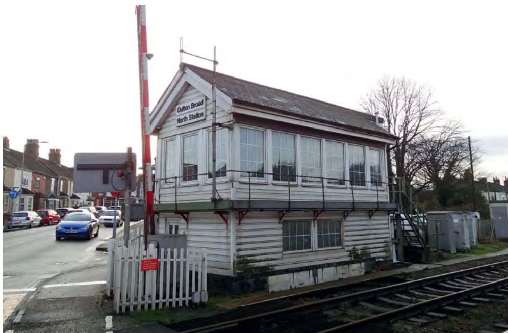
Oulton Broad North Station signal box on December 18, 2019. It was built in 1901 to a standard GER Type 7 design. The aerial on the gable end of the box is a reminder of the now defunct Radio Electronic Tokenless Block system formerly used on the East Suffolk line.
