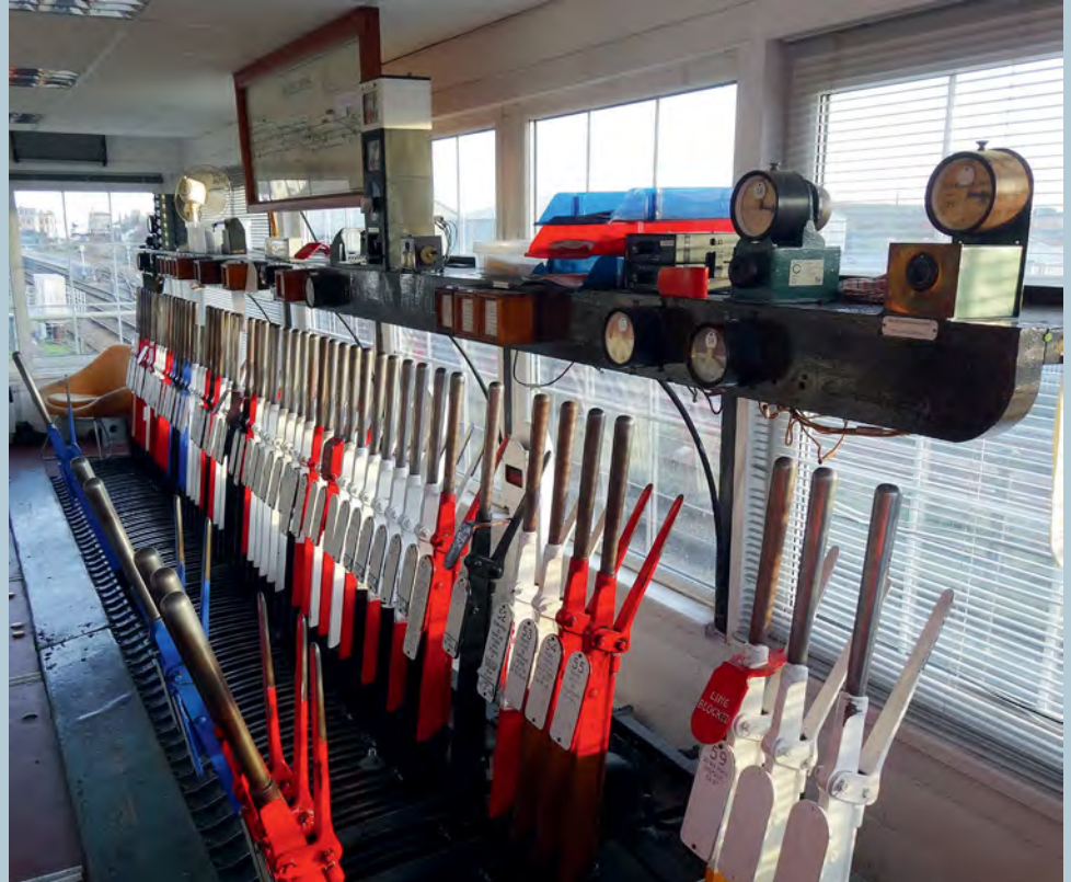
An interior view of the large operating floor of Lowestoft signal box on December 18, 2019. Most of its 61 levers were still in use when the box was decommissioned. The brass foot press studs were used to release points and facing point levers electrically.
