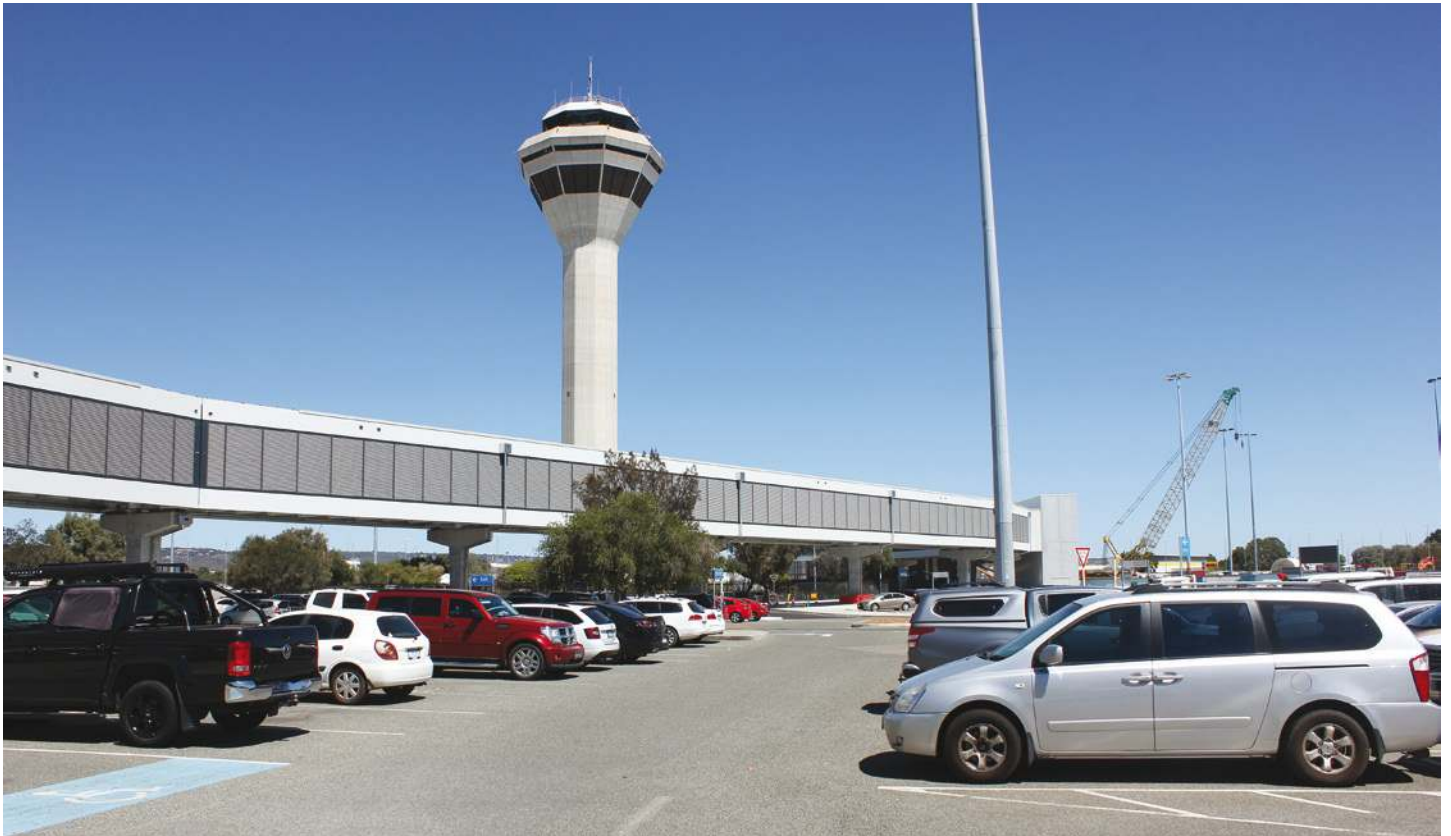
By Sunday 2 February the 'airbridge' connecting the under-construction Airport Central station to Terminal 1 at Perth Airport was substantially complete. This view looks to the station construction site. David Whiteford
