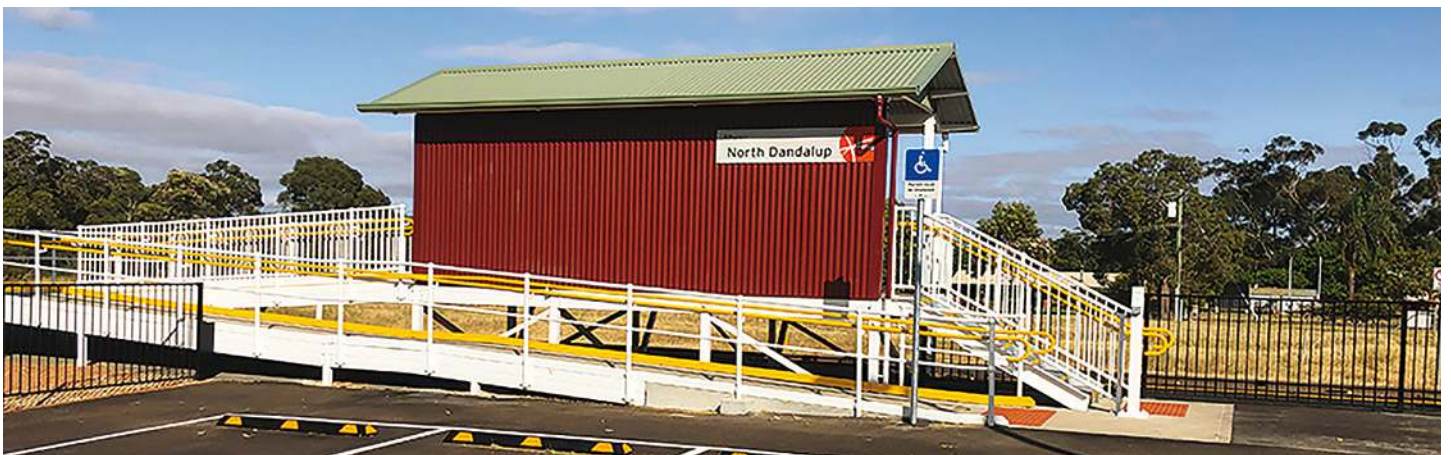
The new North Dandalup Station, viewed from the car park side. Public Transport Authority of Western Australia
