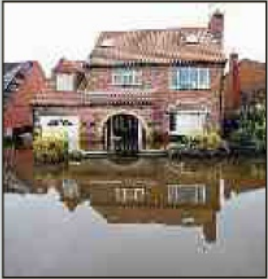
Engulfed... flood damage
