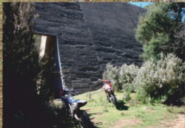
The decommissioned Mt Paris Dam, built in 1936
