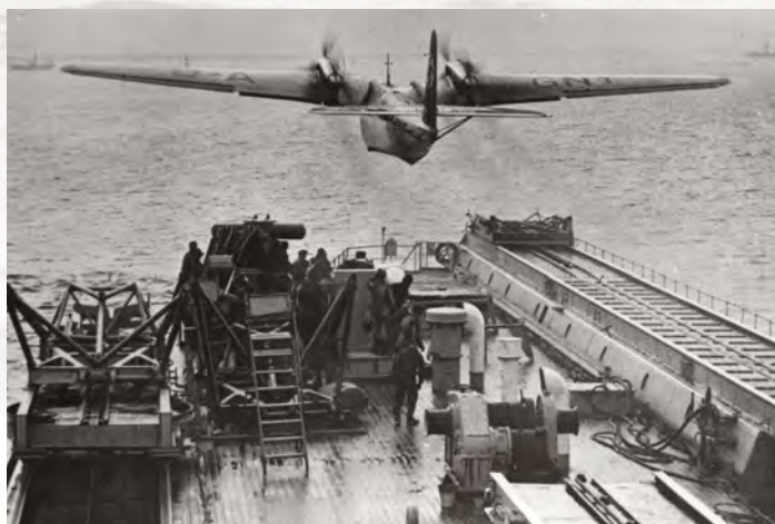
Above left: Catapult trials for the Do 26V1 on the seaplane tender Friesenland . Built for Lufthansa, the ship was used by the Kriegsmarine after 1939 and survived the war. Via Chris Goss
