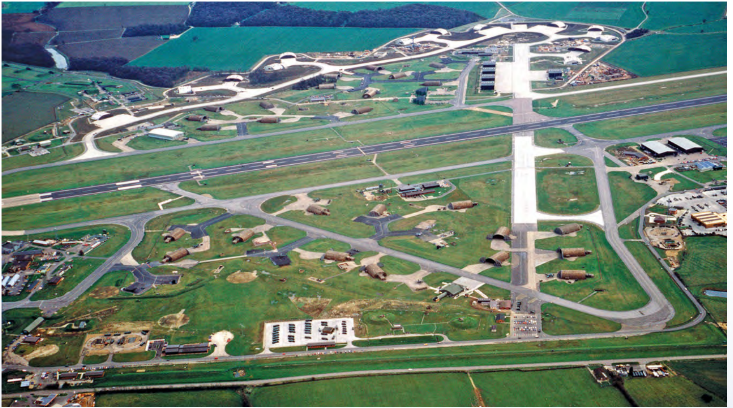
Large hardened aircraft shelters were built at Alconbury to house the TR-1s and can be seen at the top of the photo. USAF/SSgt David S Nolan
