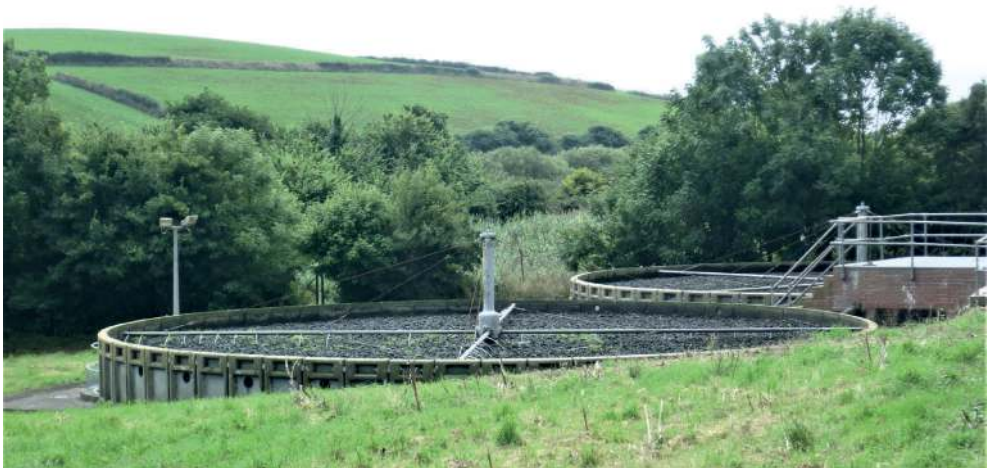
47. Filter beds at South Milton treatment works, Devon, August 2018.
