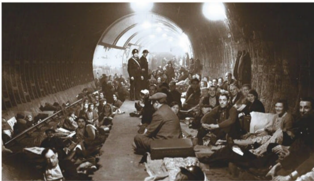
A safe-ish haven: Londoners shelter on tracks and platform alike during the Blitz
