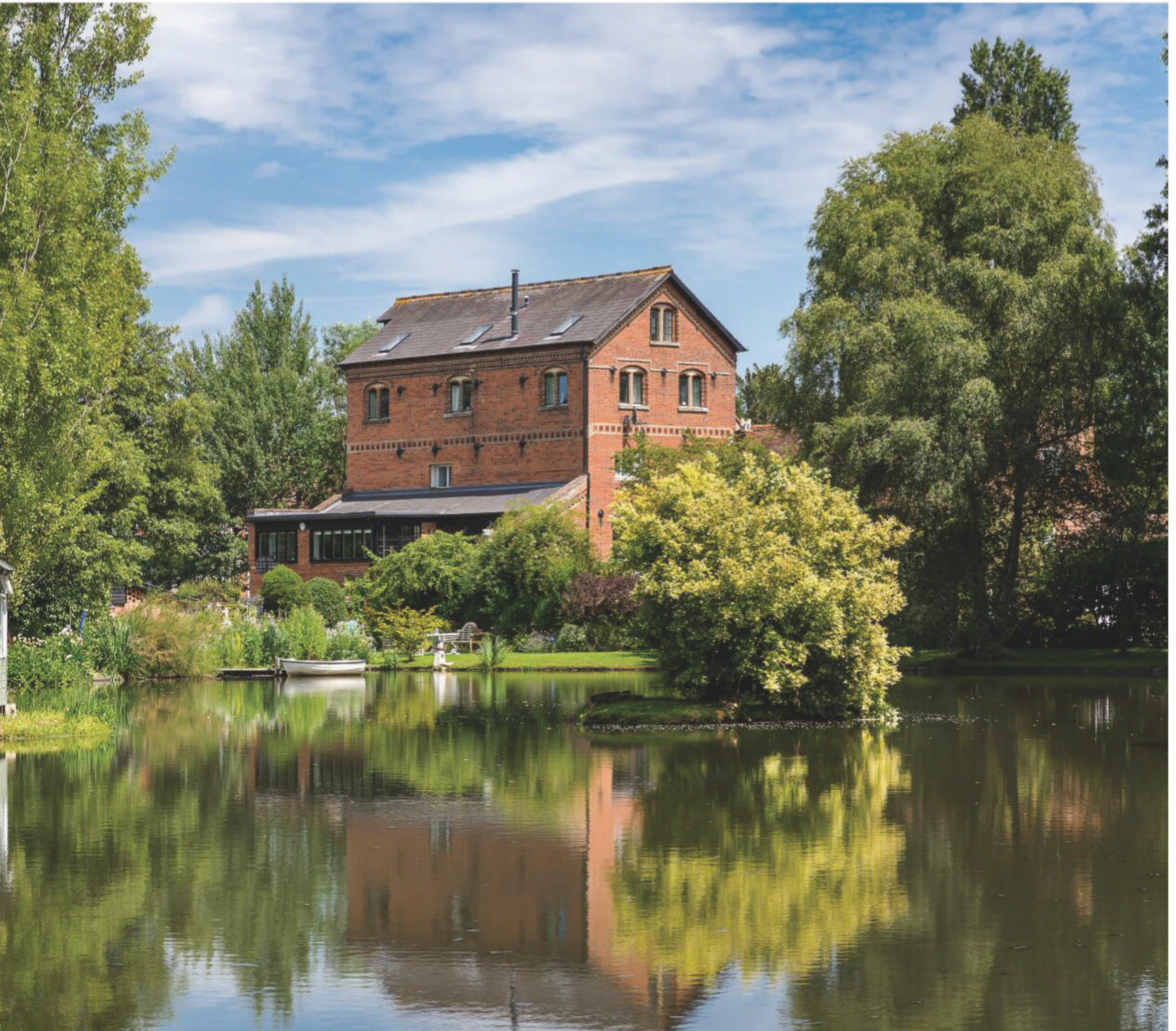
Grade II-listed Ockham Mill, completely renovated in 2015, is one of the largest former mill houses on the River Wey in Surrey. £3.5m
