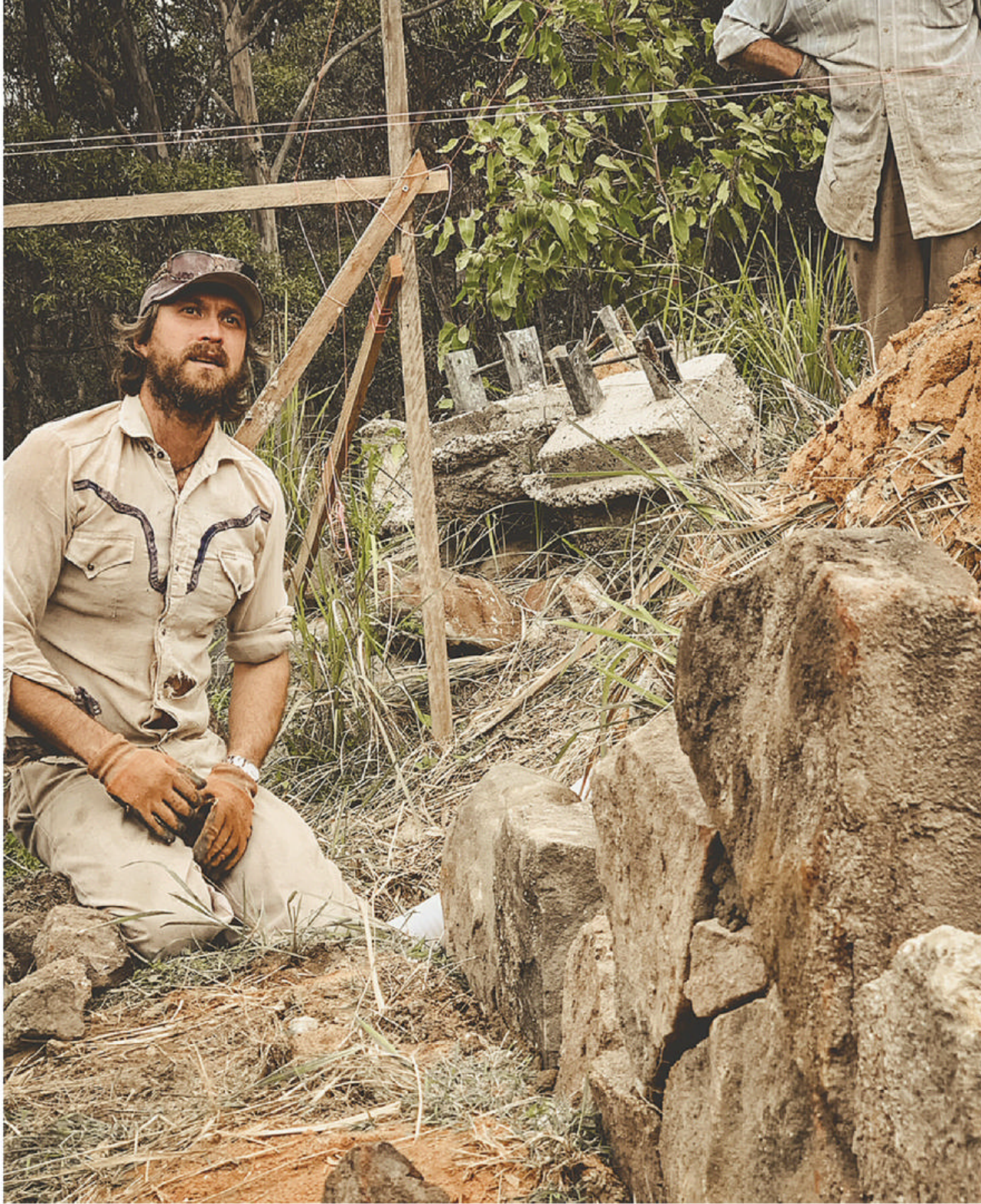
Alex down and dirty on the building site.
