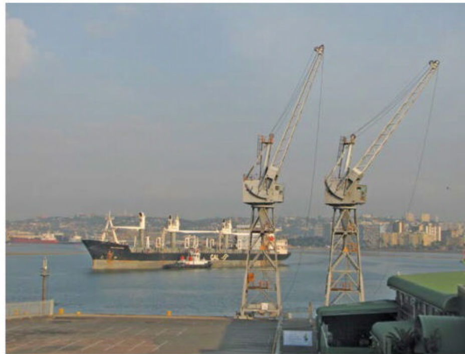
ABOVE: The Citrus Growers' Association of Southern Africa has welcomed recent steps taken at the Port of Durban to address problems with infrastructure. FW ARCHIVE
