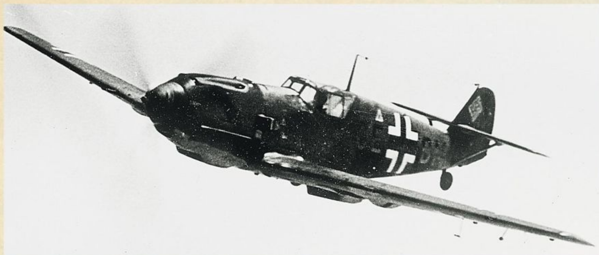
The Bf 109E was the first mass-production variant of the 109 series. By January 1940, it had displaced all previous models with 1,540 aircraft produced and 540 in Luftwaffe front-line inventory. The controls, however, became very heavy above 400mph, and this was a deficiency when it was in combat with the Spitfire, which had low, user-friendly, control maneuvering forces throughout its fight envelope. (courtesy of Warren Bodie)
