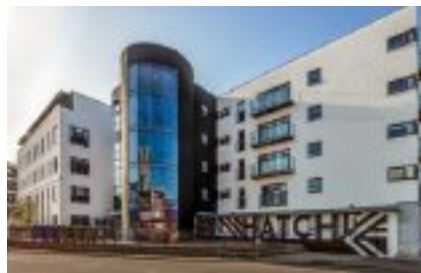
Project: Hatch Student Living, Copley St Contractor: John Paul Construction Client: Hatch Student Ventures Lead Architect: Reddy Architecture + Urbanism Contract Value: €8.5 million
