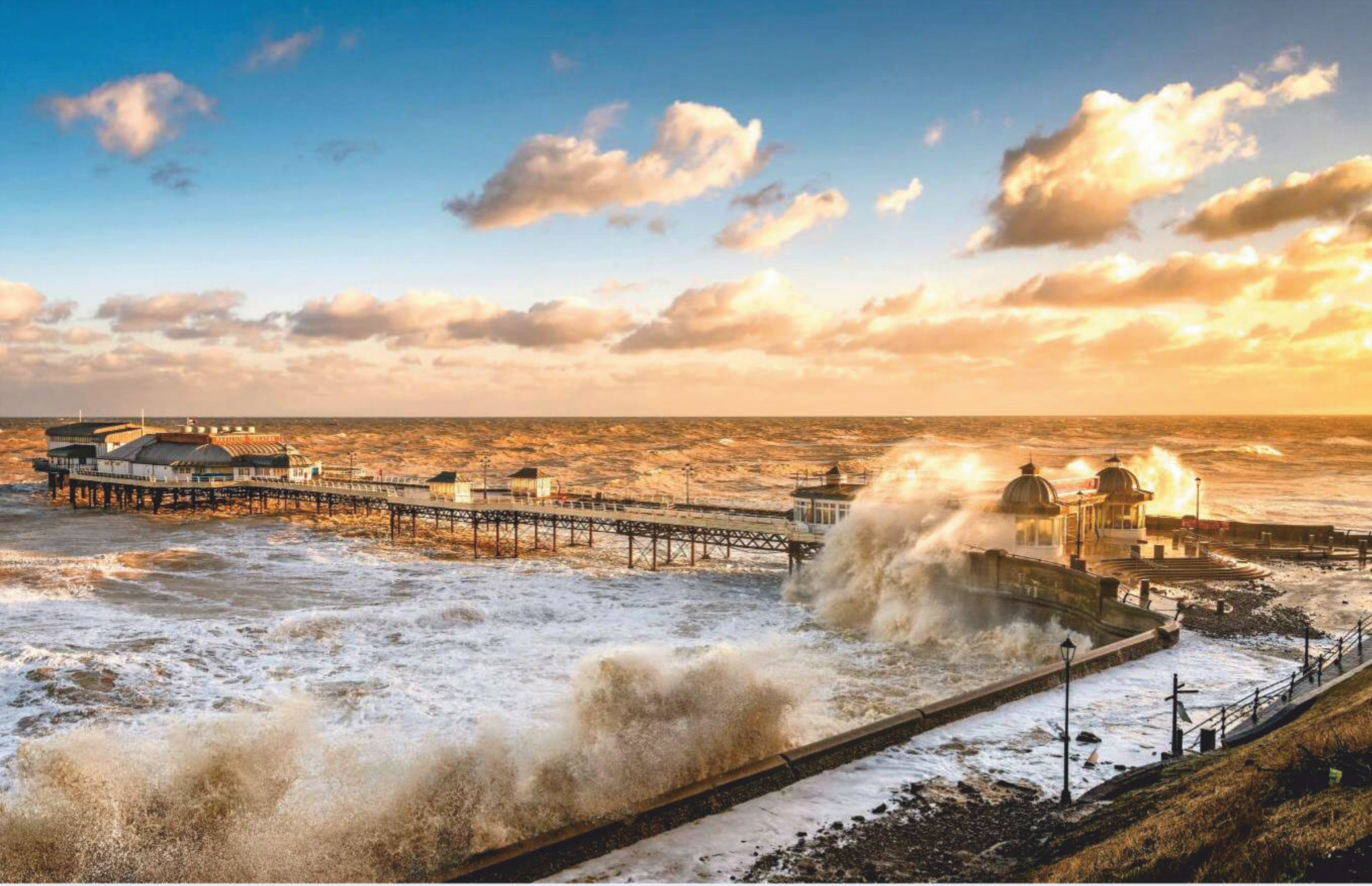
The North Sea pounds the Victorian pier and promenade at Cromer on the North Norfolk coast, in December 2013, during a storm surge. Flood defences and forecasting, however, prevented the devastating damage of the floods 60 years earlier.
