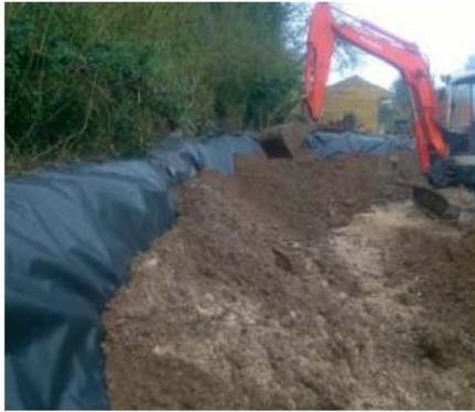
Figure 3: Knotweed Excavation with Installation of Root Barrier
