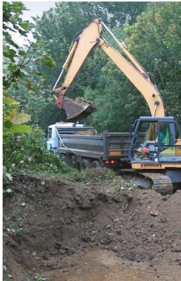
Figure 4: Dig and Dump
