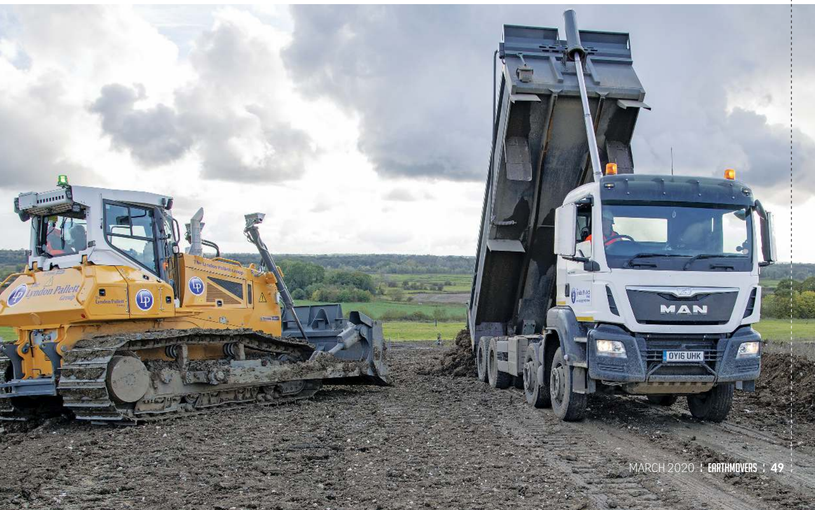
Below: The hydrostatically-driven Liebherr dozer easily managed to keep ahead of the constant stream of trucks delivering inert soil.
