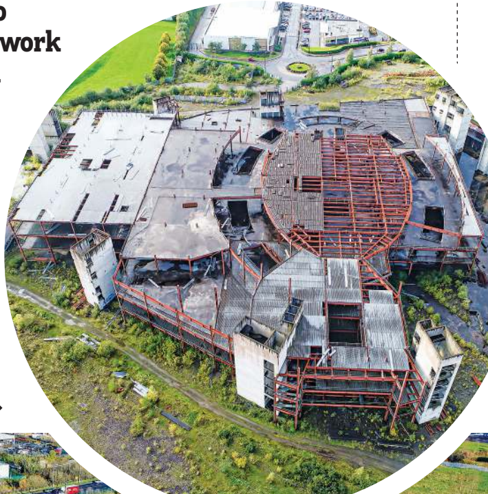
The long abandoned construction of the 10-acre Parkway Valley shopping centre site left imposing steel and concrete structures to be removed.
