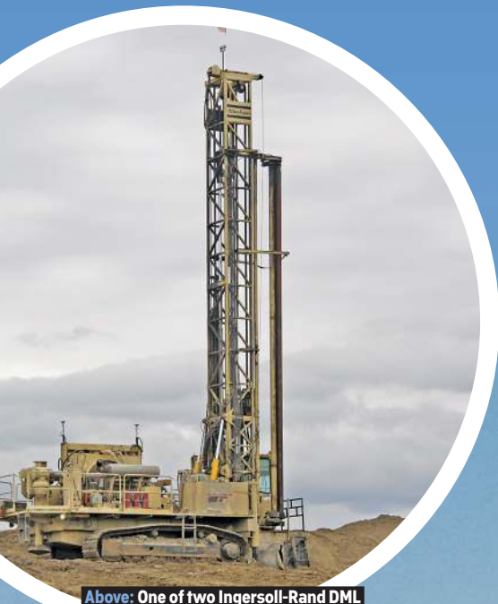
Above: One of two Ingersoll-Rand DML blast hole drills are employed to drill some hard, rocky areas encountered in the overburden.
