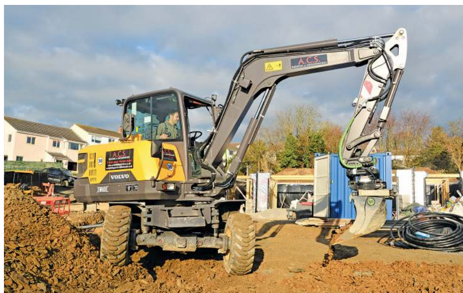
Top and above: The wheeled machine was driven to site under its own steam and proved to be particularly suitable for manoeuvring around the tight spaces on this building plot.
