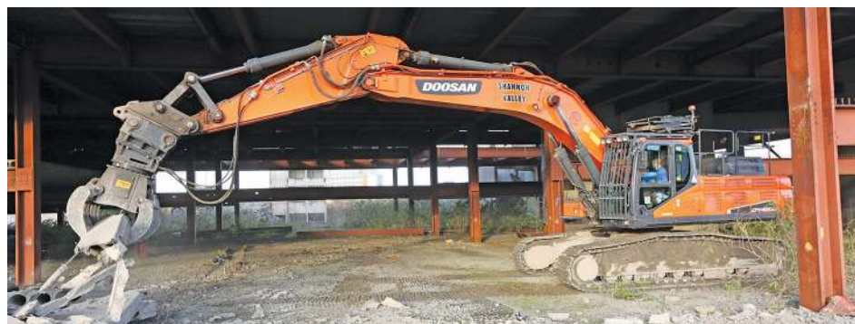
Above and left: A number of Doosan excavators are also in the Shannon Valley fleet, the DX420-5 performing a number of key roles around the site.
