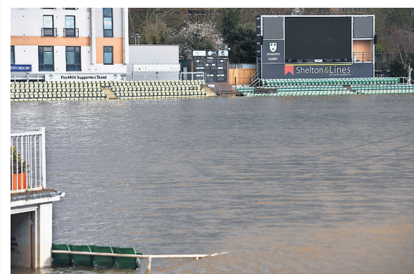
◀ New Road, always flood-prone, has spent 66 of the past 131 days under water
