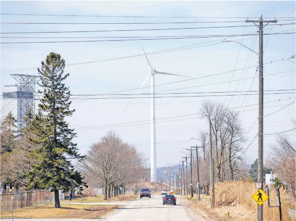
A wind turbine is seen at the Pickering Nuclear Power Generating Station near Toronto last April. Ontario's Independent Electricity System Operator recently released its annual planning outlook, which shows continued surpluses in the amount of energy we have the capability to produce. CARLOS OSORIO/REUTERS
