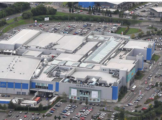
It is hoped that east-bound traffic queues near Mahon Point shopping centre for the Jack Lynch tunnel would be relieved by an interchange that has been dogged with issues since it was first announced.
