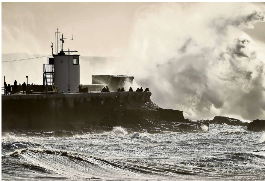
With floods and storms on the increase across these islands a collision with reality cannot be postponed.
