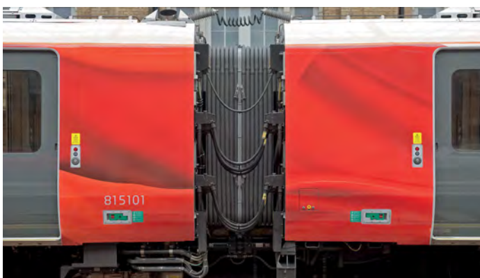
Resolution agreed: the ladder arrangement of cables seen here on Azuma No 800101 is to be modified for safety reasons. Tony Miles
