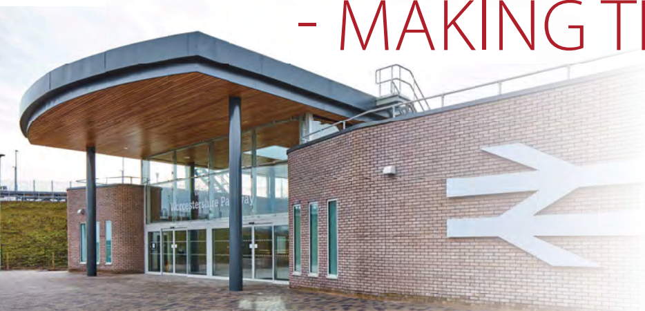
Worcestershire Parkway is the first new station to be opened in the county for over 100 years. The station was developed and delivered by Worcestershire County Council with the support of SLC Rail.
