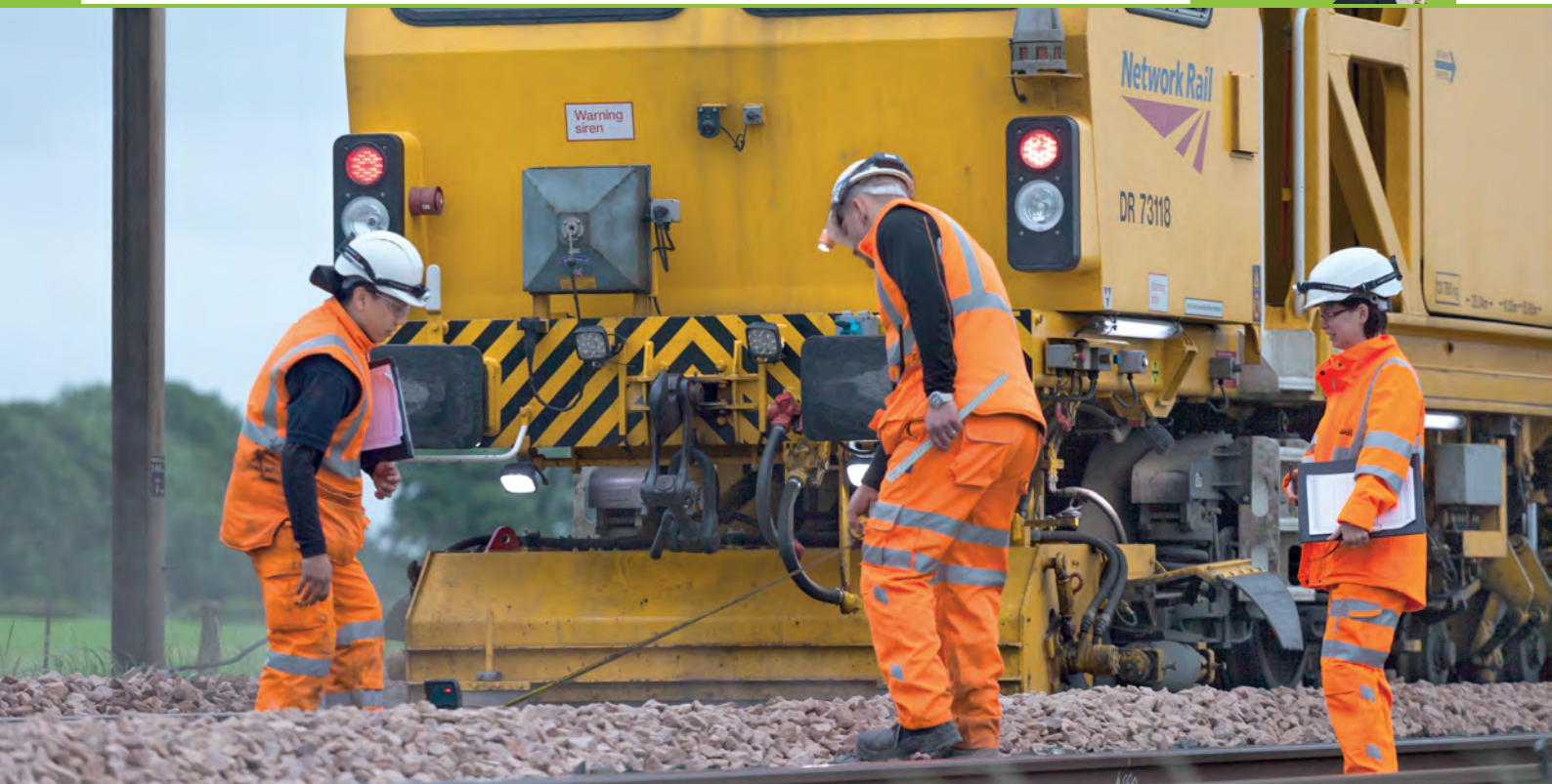
Making a good ballast bed: tamper at work at Brock on the West Coast main line on 21 June 2015. Rob France
