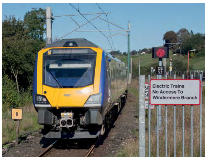
New train but no wires: Northern's No 195102 runs onto the Windermere branch at Oxenholme on 2 October 2019 with the 11.28 Manchester Airport to Windermere. Class 331 EMUs fitted with batteries are proposed to take over these services. Tony Miles
