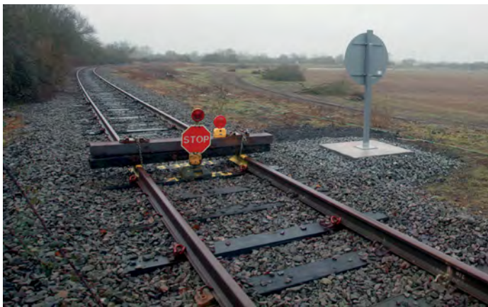
Preparing for HS2: looking north towards Claydon Junction on 22 January 2020, showing the area now given over to HS2 works. Phil Marsh
