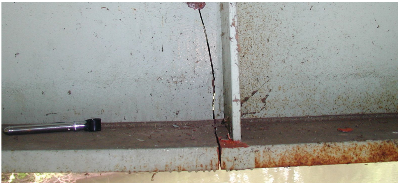
above: A close-up of a fracture-critical-designated girder on the U.S. 422 Bridge over Schuylkill River. The bridge continued to carry service loads in the failed condition before the fracture was discovered and repaired.
