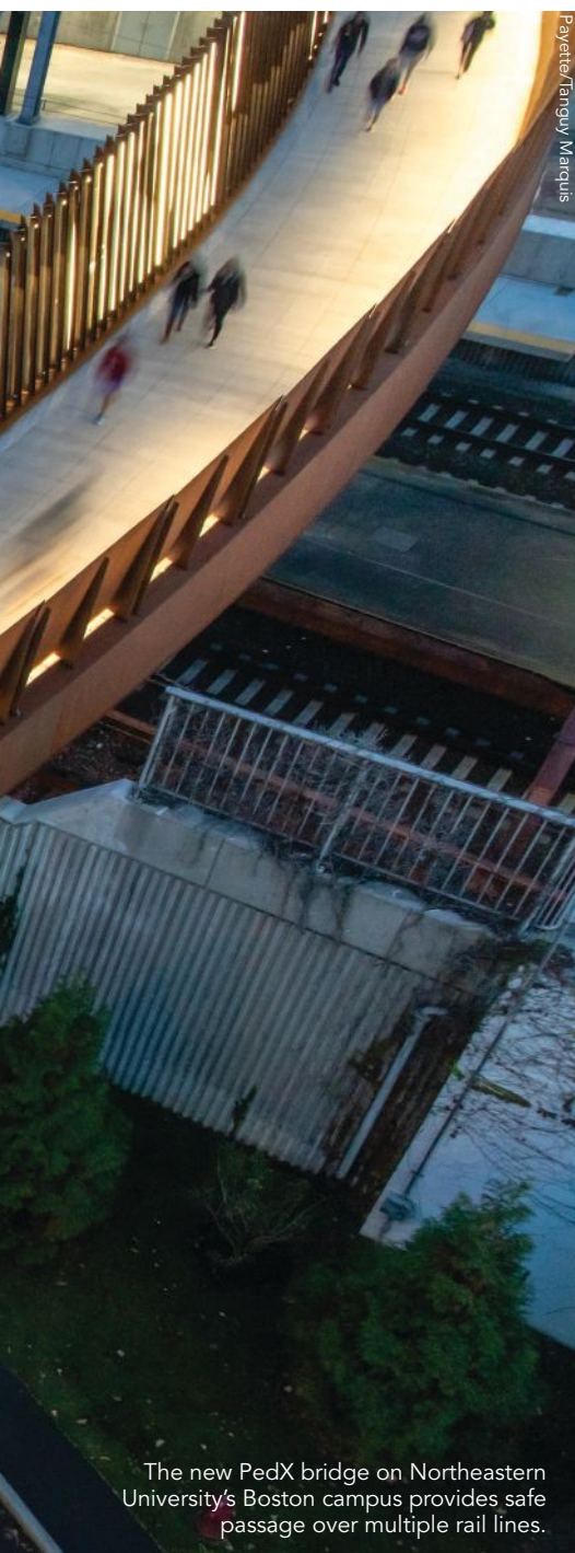
Weathering steel panels protect the train tracks and adjacent power lines from pedestrians and vice versa.
