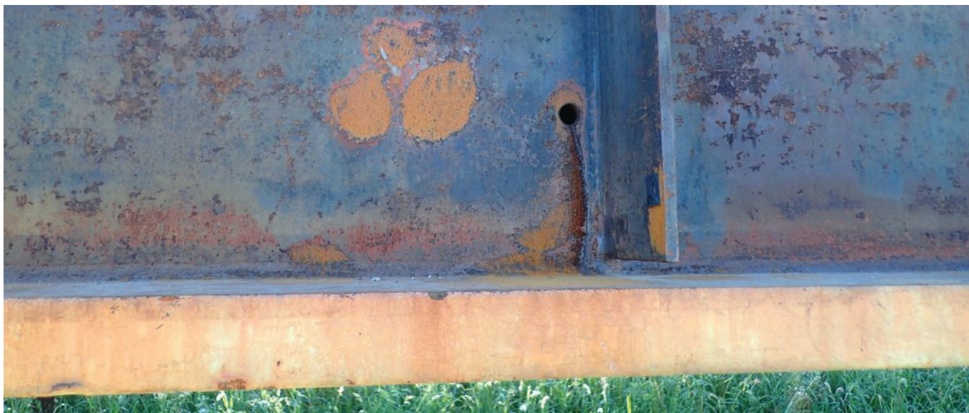
above: A close-up of a fracture-critical-designated girder on the U.S. 422 Bridge over Schuylkill River. The bridge continued to carry service loads in the failed condition before the fracture was discovered and repaired.
