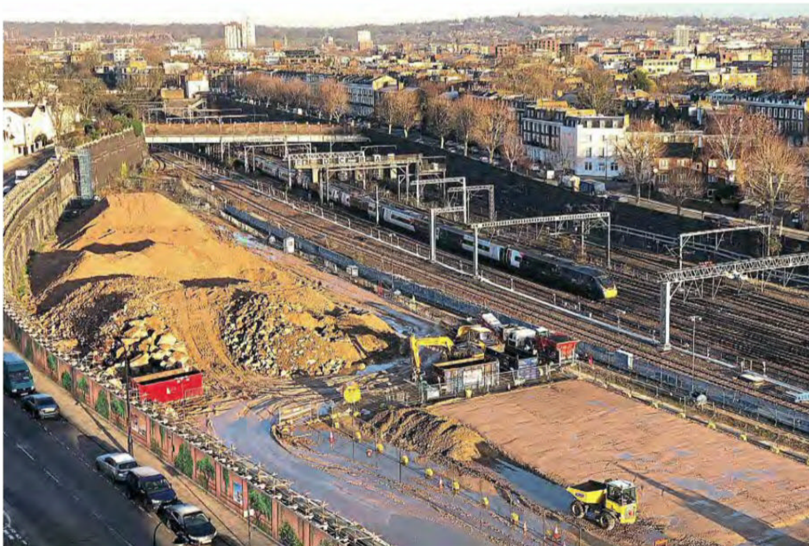
An Avanti 'Pendolino' arrives at Euston on January 18, past the site of the former Downside Carriage Shed, which is now being used as a HS2 worksite for crushing and removing spoil created by the demolition of other acquired properties in the area. Steve Morris
