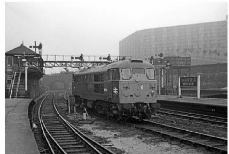
The former signal box at the north end of platform 1 in October 1969, as Class 31 No. D5543 (later 31125) waits in the centre road for its next duty. Rail-Online
