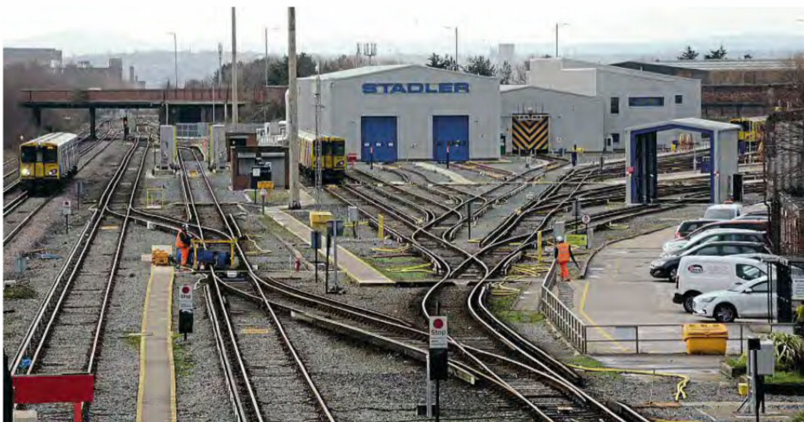
A view of Kirkdale station looking south from the adjacent station. The new buildings were completed at the end of 2019 and comprise (from left) the two-road servicing shed, the single road maintenance and wheel lathe building, and the office block. Siding space is off to the right where the previous now-demolished shed was.
