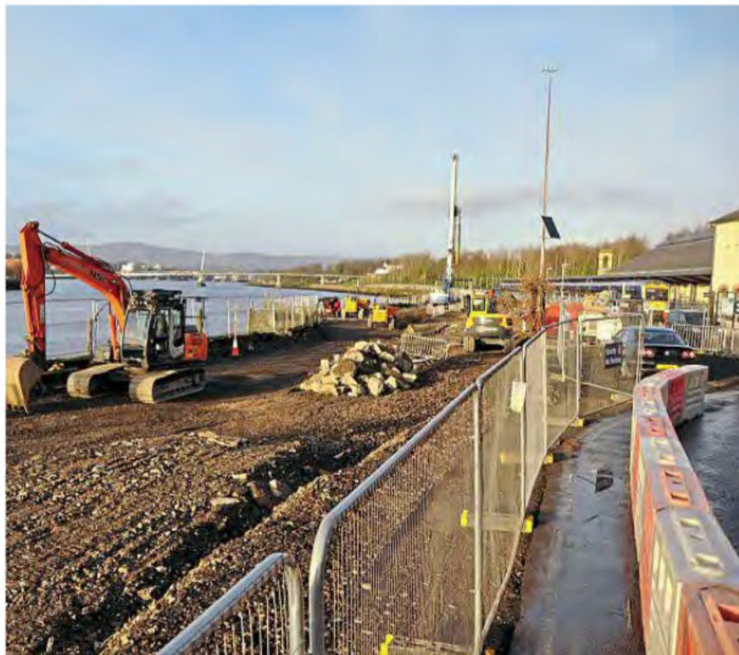
LONDONDERRY REBUILD: The last remnants of the 1980-built terminus are being cleared in preparation for the site to be a car park and bus turning circle. This January 26 view shows a 3000 Class DMU at the refurbished Waterside station in the background. Chris Playfair
