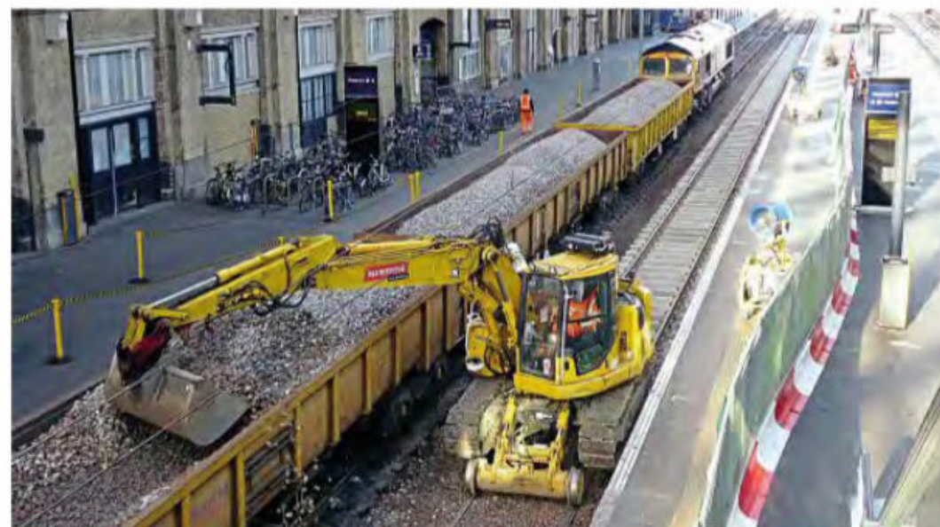
King's Cross was closed on January 18/19 for track renewal and ballasting work, leading to the rare sight of engineering trains in the London terminus. This view shows ballast being unloaded from a train headed by GBRf's No. 66708 on the first day. Bill Bass
