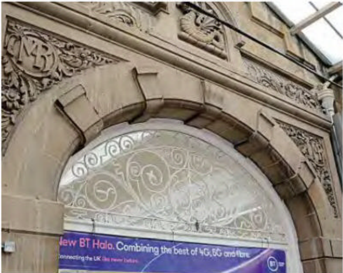
Architectural detail illustrates the station's Midland Railway origins in Victorian times.
