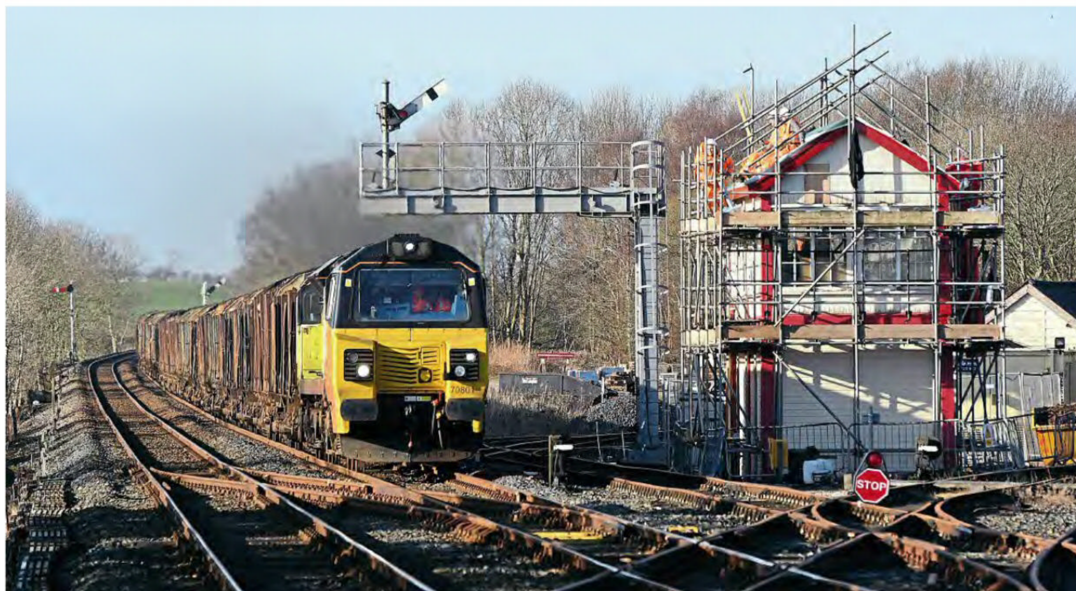
APPLEBY BOX UPGRADE: The 1950s signalbox at Appleby, Cumbria, has been upgraded to extend its working life into the 2050s, work that required it to be switched out from mid-November to mid-January, creating a long section from Kirkby Thore (British Gypsum) to Kirkby Stephen. The work should be fully completed in early March, and then will mean semaphore signals can be enjoyed on this part of the Settle & Carlisle line for the next three decades. Colas' No. 70810 passes the box on February 6 with the 6J37 Carlisle to Chirk log train. Mike Summers
