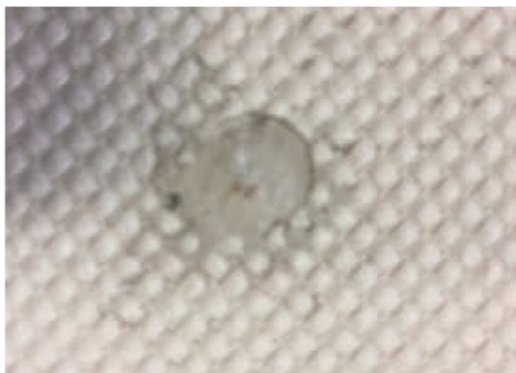
The top of the epoxy putty repair.
