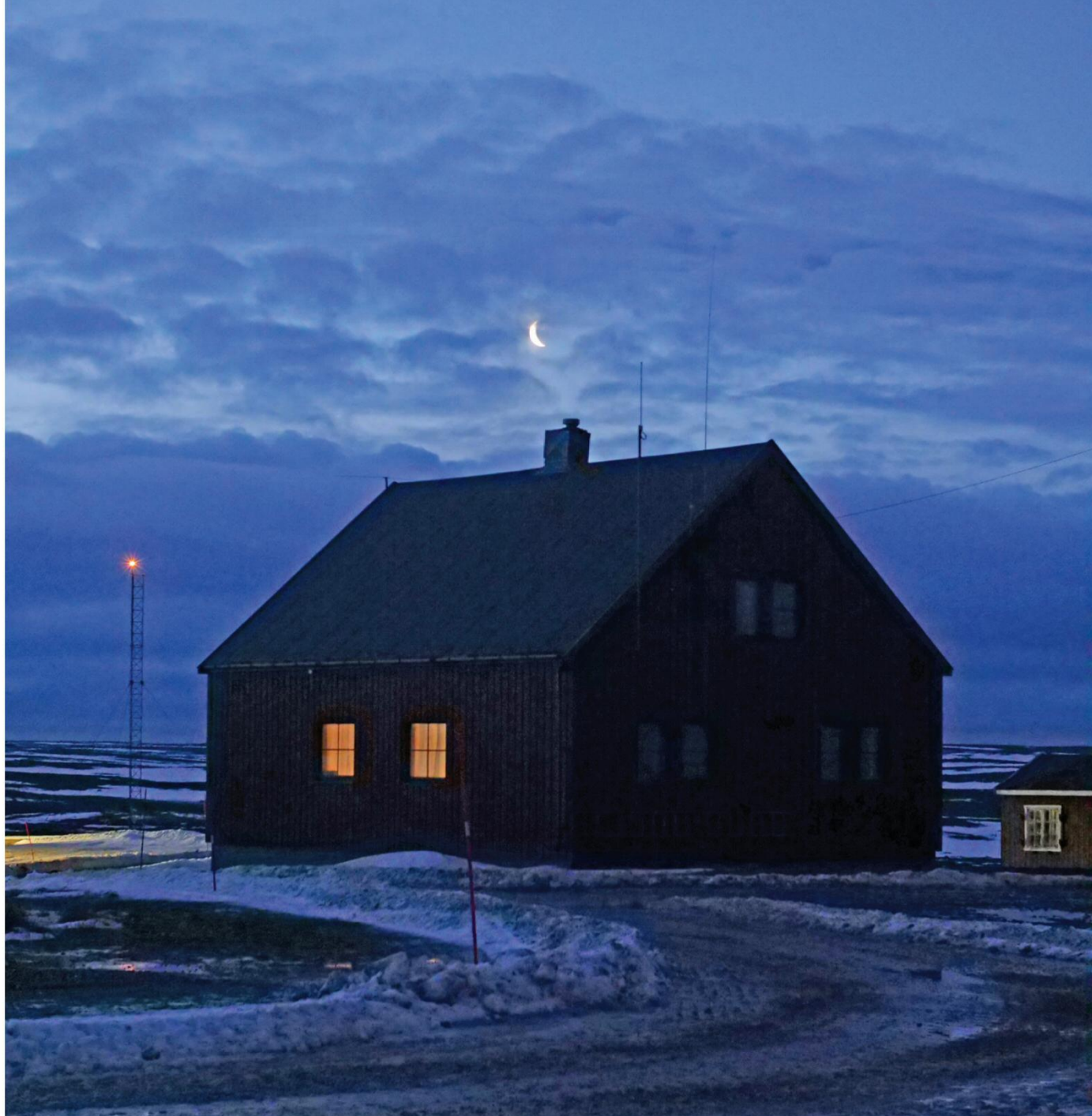
A bunkhouse at the meteorological station in Bjørnøya, an island near the western edge of the Barents Sea
