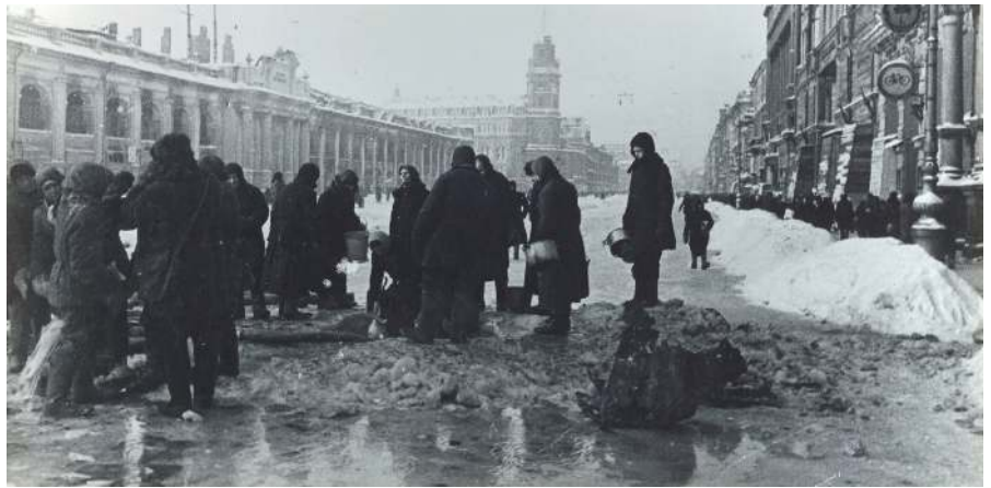
After the German aerial bombing destroyed the public works infrastructure, the citizens of Leningrad were left without drinking water and all other life-sustaining essentials
