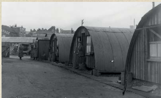
Above: Nissen Hut accommodation of the FANY/VAD St. Omer Convoy
