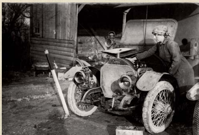
With overall and headscarf donned for protection, this FANY member services her Napier vehicle's engine
