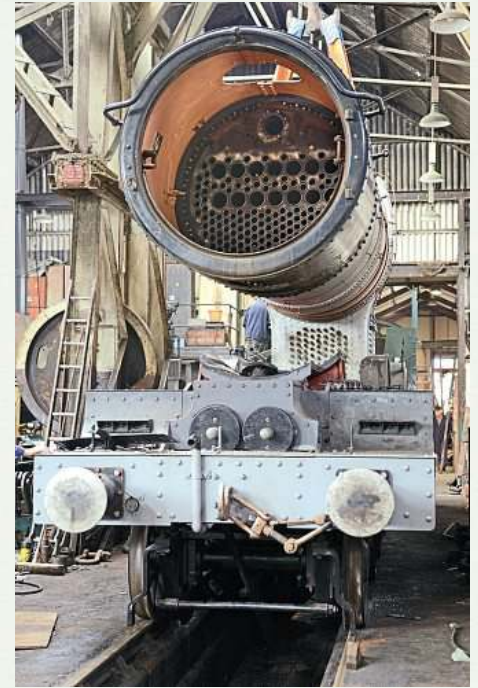
The boiler of No. 4079 is carefully craned onto the frames in October 2015.
