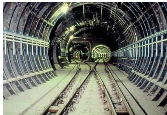
The newly installed points at the Prudhoe Street crossover beneath Newcastle. NEXUS
