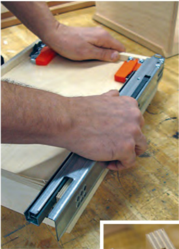
Once the locking devices were installed, marking a centerpoint in the drawer back for the slide's hook was a simple matter of engaging the slide hardware and bumping the hook against the drawer back (top inset). Drill the 1/4"-dia. hook holes 13/32" deep (bottom inset).
