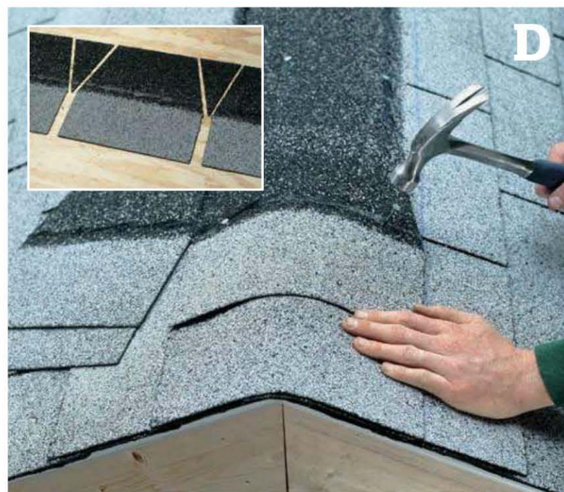
Divide the shingles into thirds , then trim the corners to create the shingle caps (INSET). Install the caps at the ridge.
