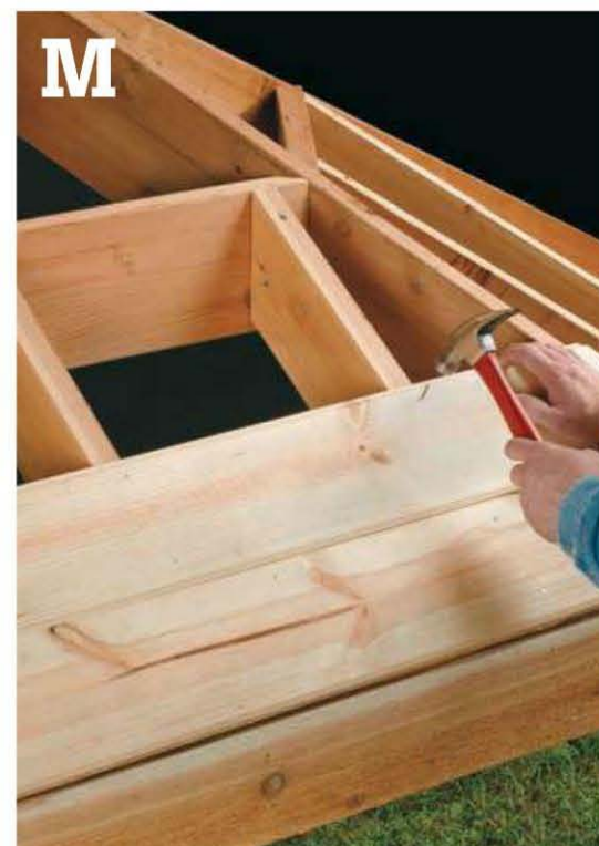
Miter the ends of the sheathing boards and make sure the tongue-and-groove joints are tight before nailing.
