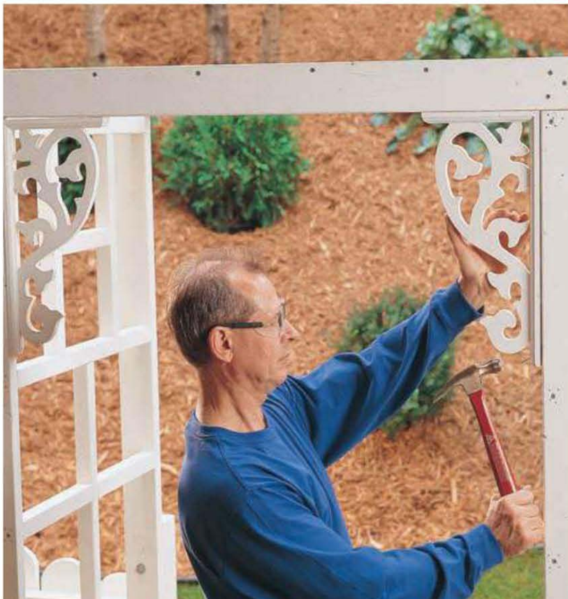
Add millwork brackets at each corner where the tie beams and the trellis frame posts meet. Secure with finish nails.
