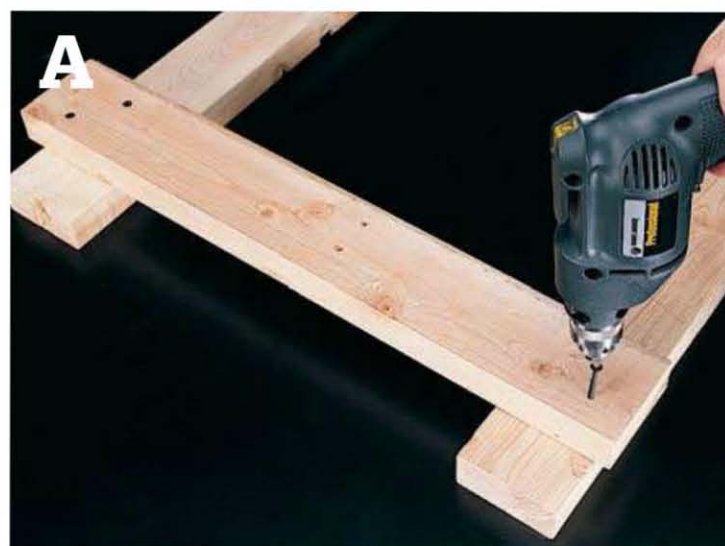
Cut the batter board pieces from 2 \times 4 lumber and assemble them with screws.
