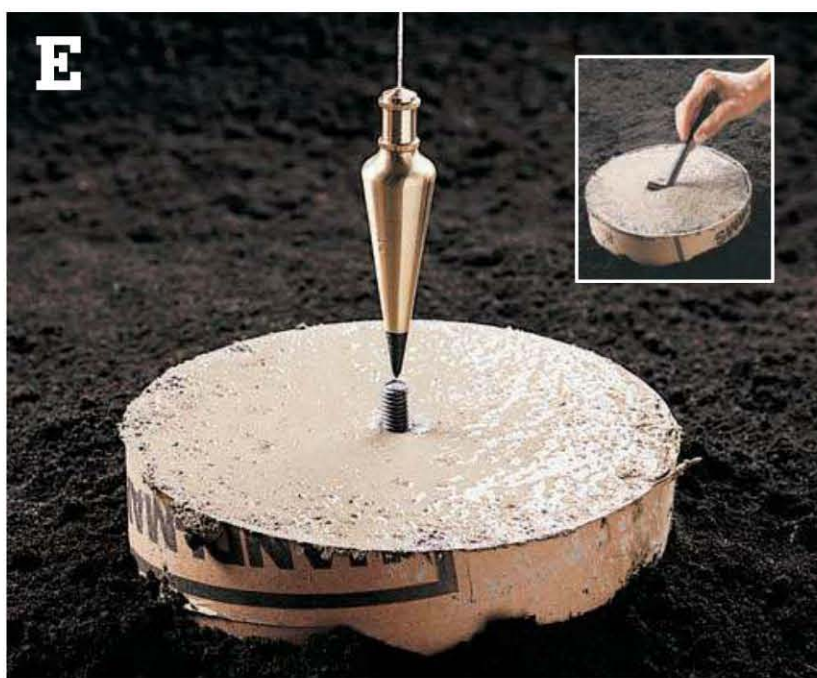
Fill the forms with concrete, then set the J-bolts (INSET). Check with a plumb bob to make sure the bolts are centered.
