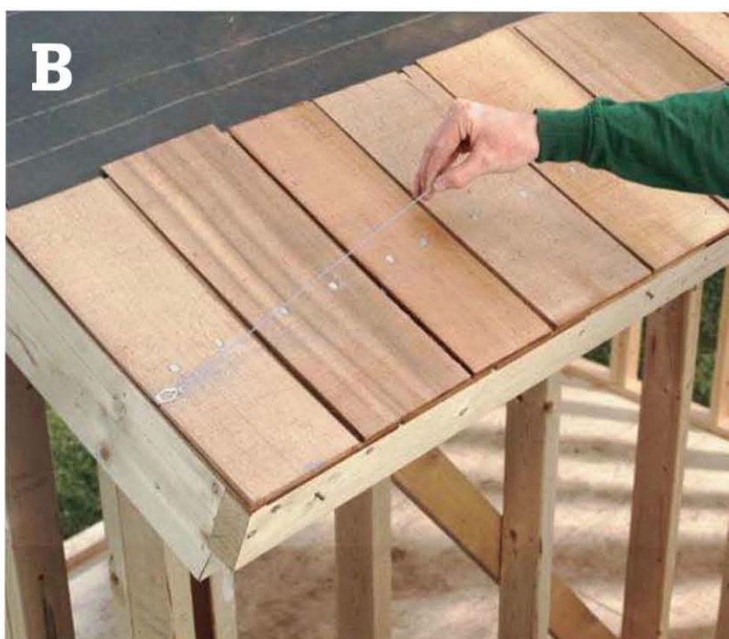
Install the first course of shingles on top of the starter course, offsetting the shingle gaps 1½" between the courses.
