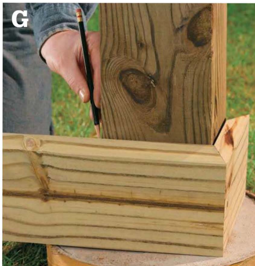
Hold together the mitered ends of two trim boards and mark the uncut ends along the post.
