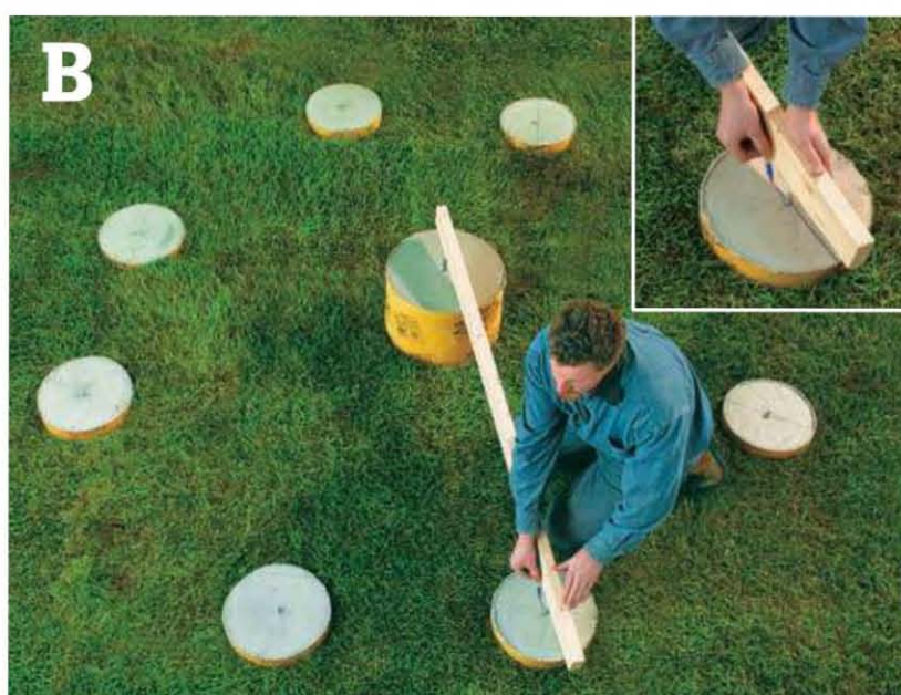
Set a board across the center and each outer footing and mark a line across the top of the outer footing.
