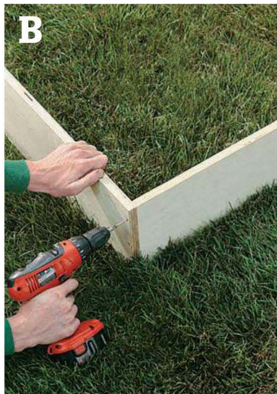
Assemble the form pieces with 2½" deck screws, then check the inner dimensions of the form. For long runs, join pieces with plywood mending plates.
