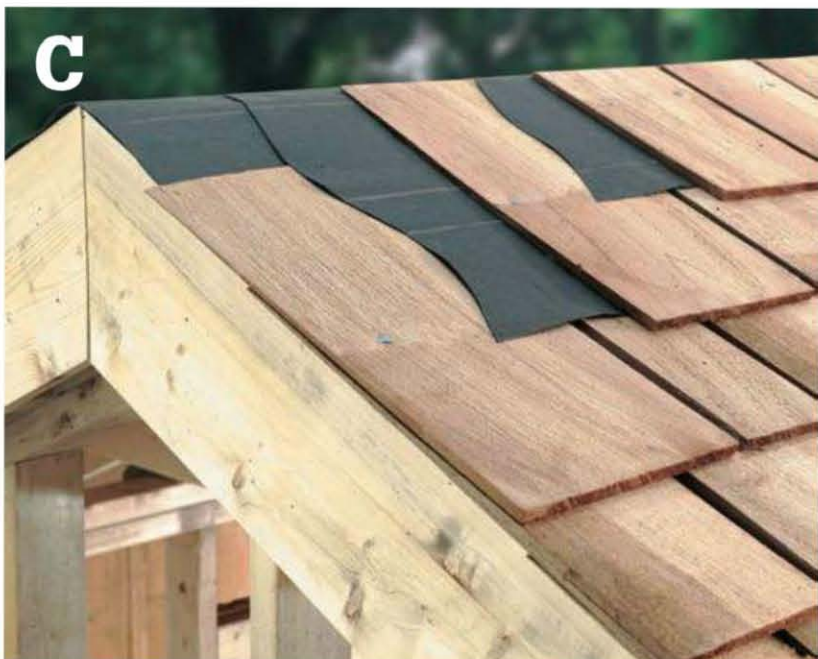
Cover the ridge with 24" of building paper, then a course of trimmed shingles. Repeat with 12" of paper and shingles.
