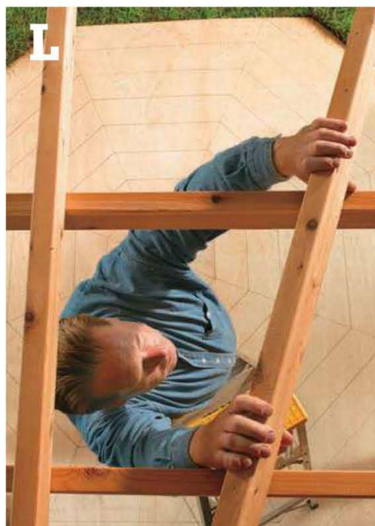
Install the collar ties so that the upper pair rest on top of, and are perpendicular to, the lower pair.
