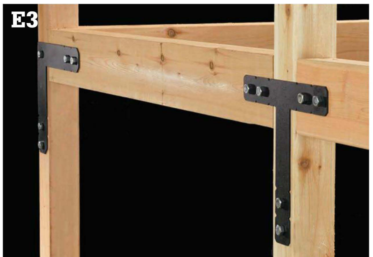
Side wall beam to corner post connection.
