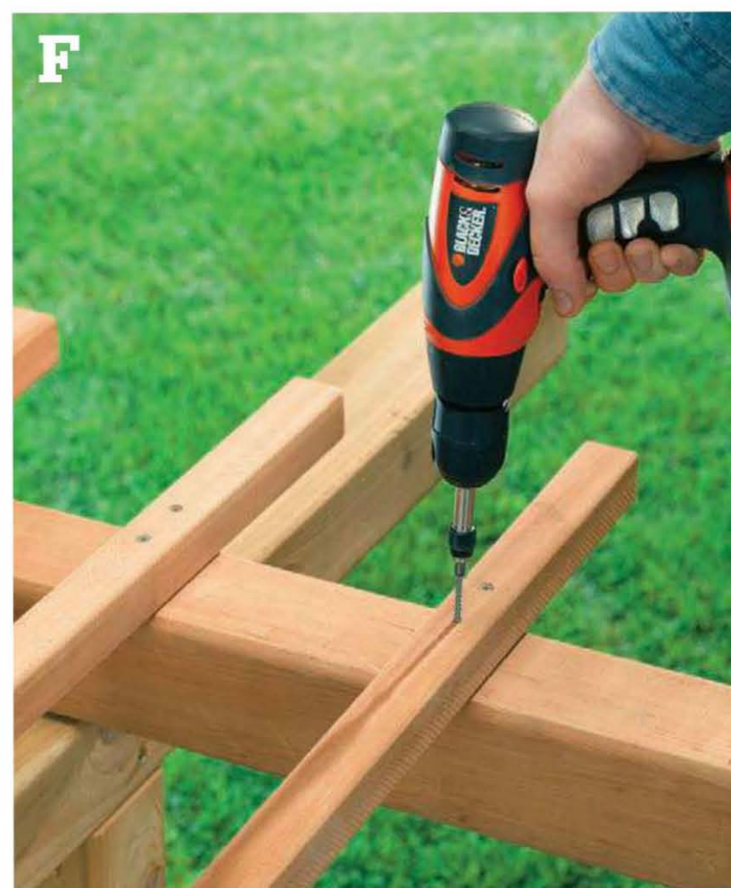
Install the upper beams and slats using the same procedure for securing the lower beams and slats.
