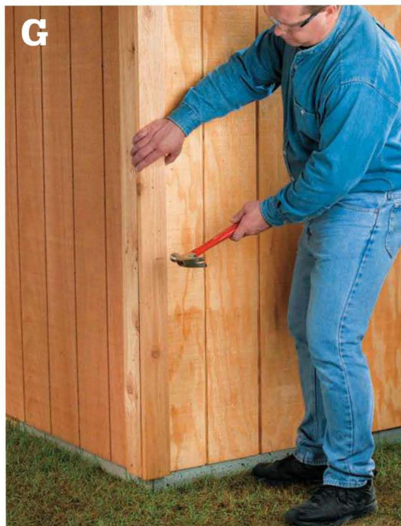
With the exception of the top cap trim , install the trim so all of the joints are flush.
