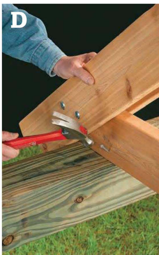
Install the trusses by toenailing through the truss bottom chords and into the beams.
