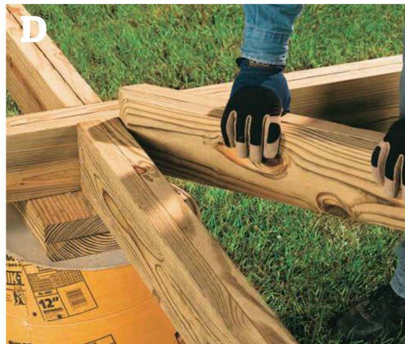
Miter the ends of four of the double joists so they meet flush with the full-length joist and those perpendicular to it.
