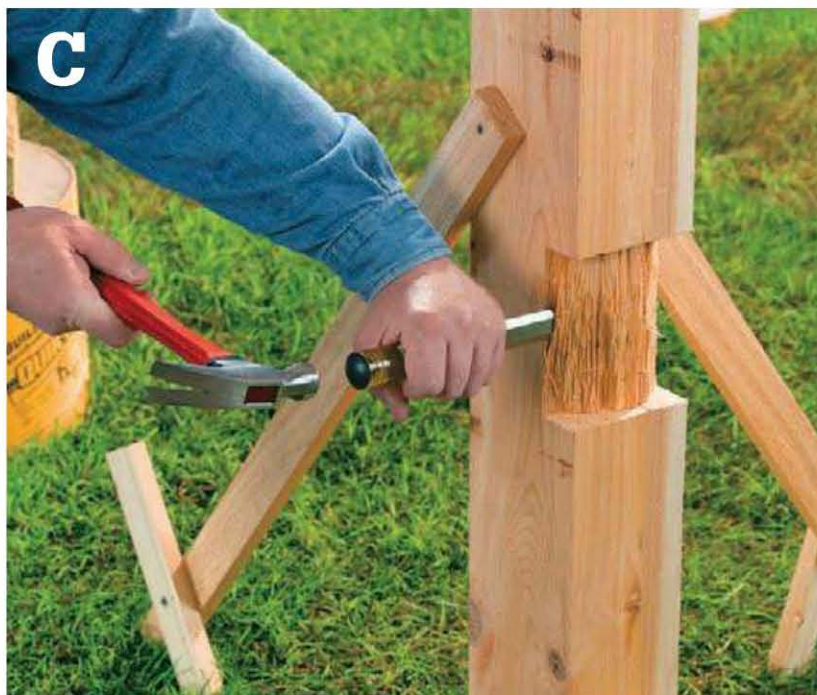
Cut the post notches by making horizontal cuts with a handsaw or circular saw, and then remove the remaining material with a chisel.
