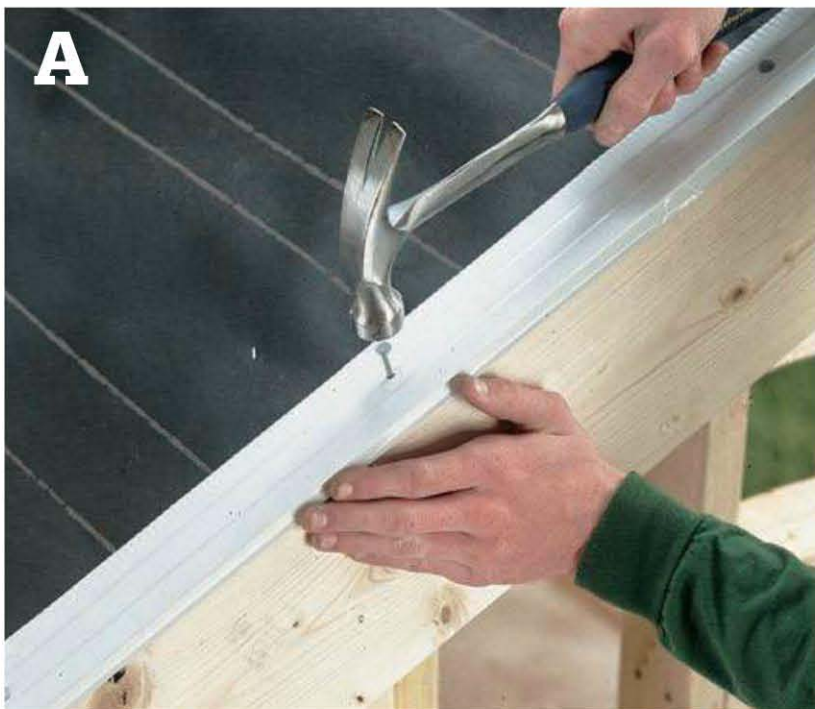
Install drip edge along the eaves over the sheathing. Add the building paper, then install edging along the gable ends.
