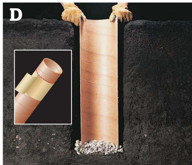
Wrap paper around the form to mark a straight cutting line (INSET). Set the forms in the holes on top of the 4" gravel layer.
