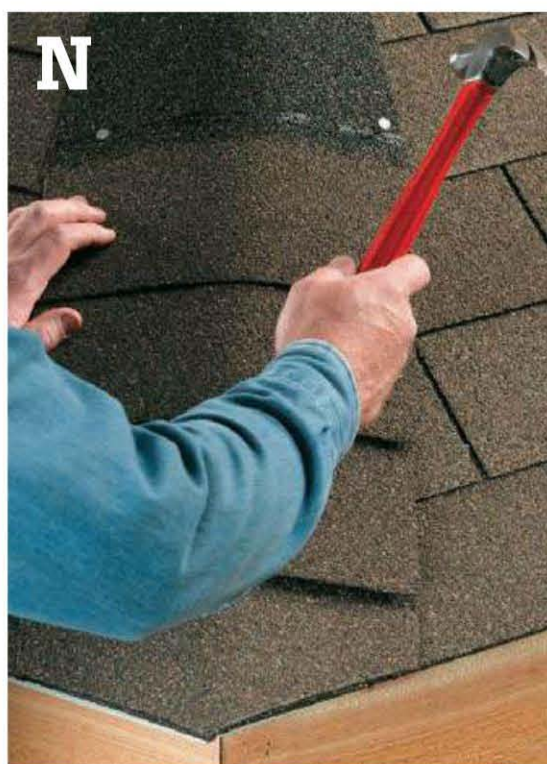
Shingle the roof sides individually, then cover the hip ridges with caps, overlapping the shingles equally on both sides.
