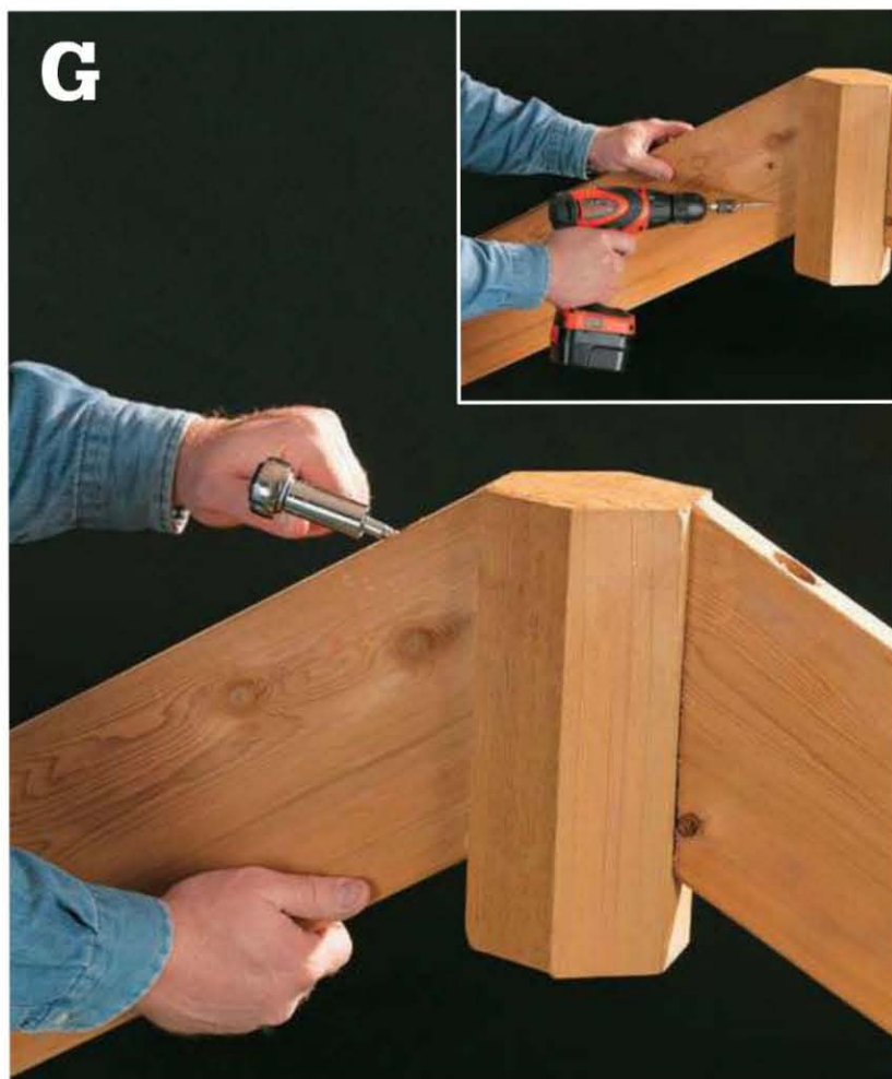
Install the hip rafters so their top ends are flush with the top of the hub. INSET: Toenail the rafters to the sides of the hub for extra support.
