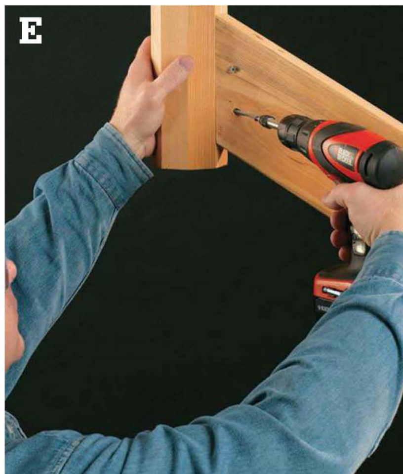
Drive angled screws to fasten the rafters to the roof hub.
