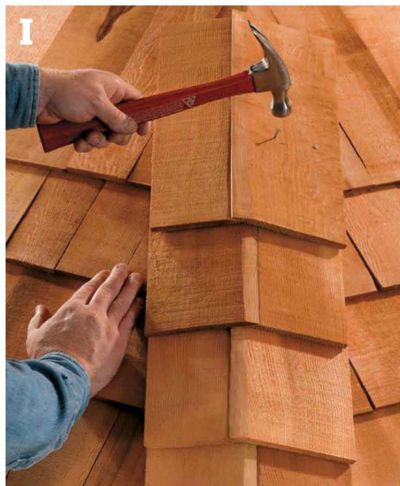
Bevel the edges of both shingles for each cap, and alternate the overlap between courses.
