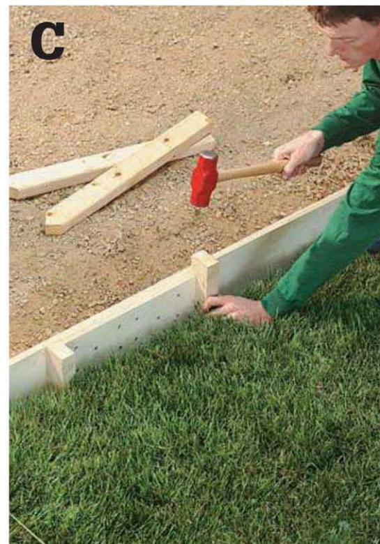
Drive stakes every 12" to support the form, using the mason's lines to make sure the form remains straight.
