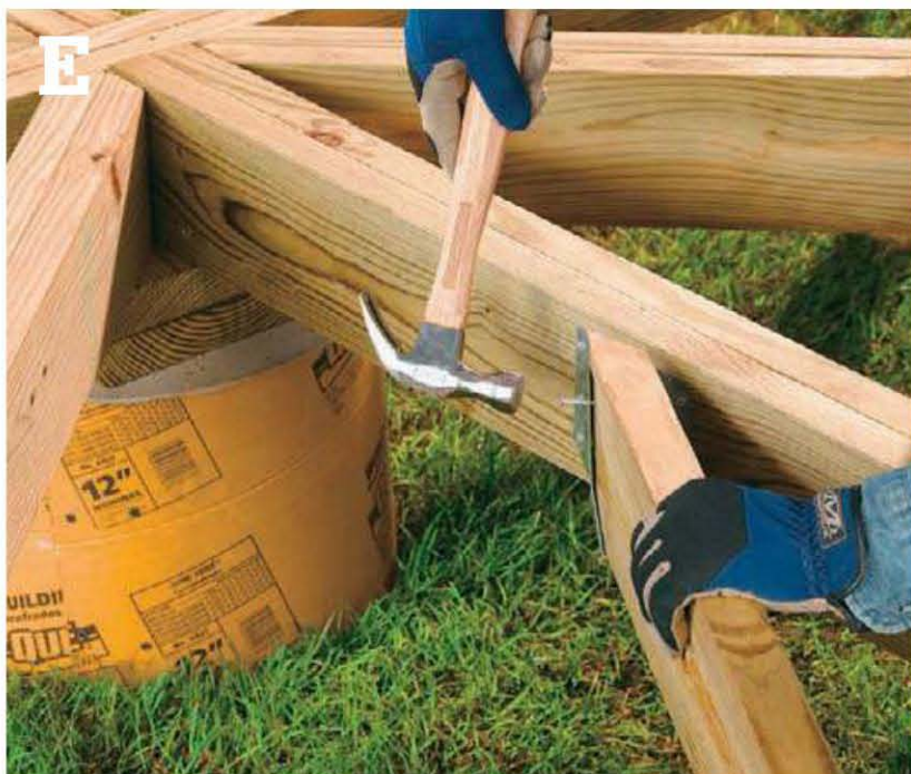
Fasten the angled floor joists to the sides of the double joists with skewable metal anchors.
