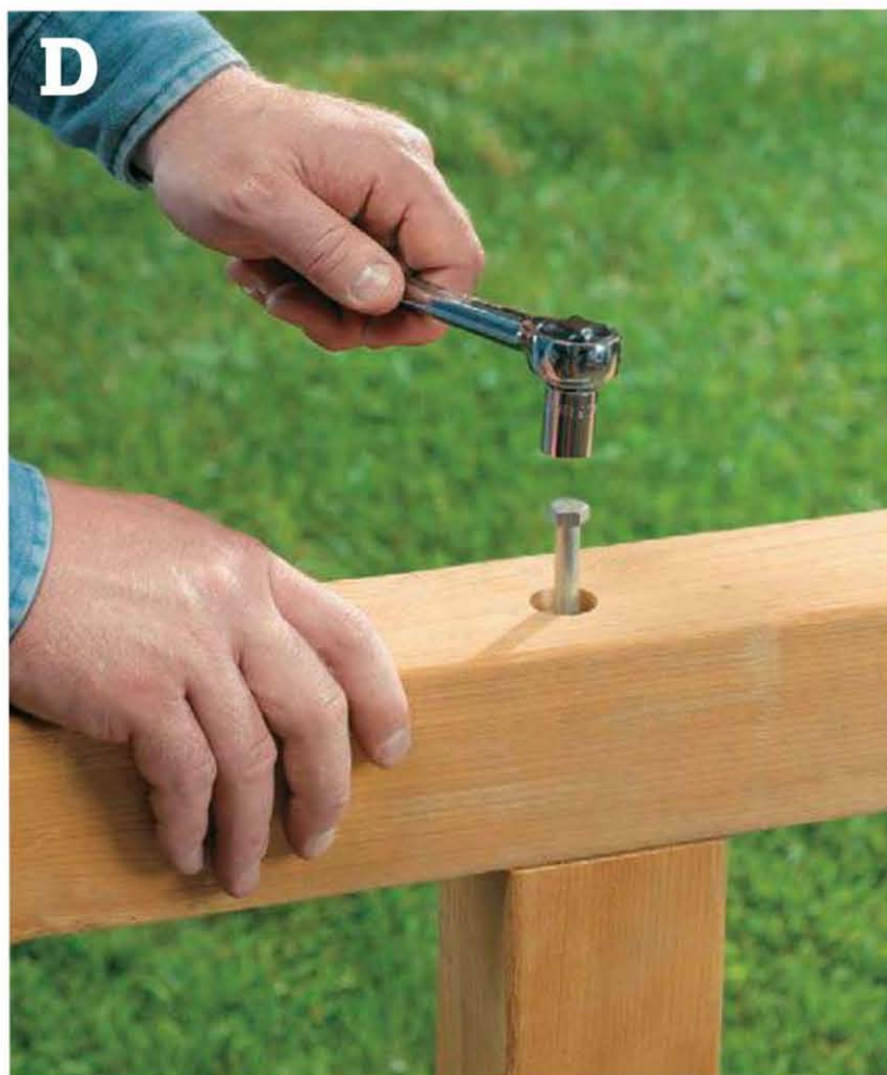
Test-fit the main beams to the posts, then drill counterbored pilot holes and fasten the beams with lag screws.
