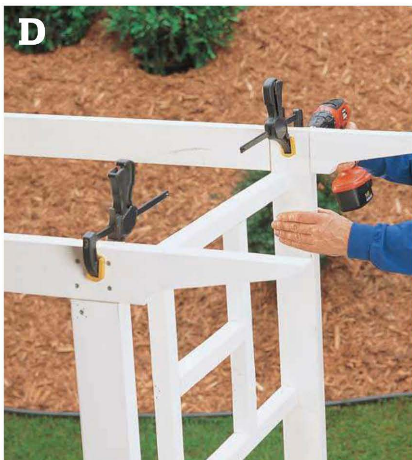
Clamp the tie beams to the trellis posts, then attach with five 1¼" corrosion-resistant deck screws at each joint.
