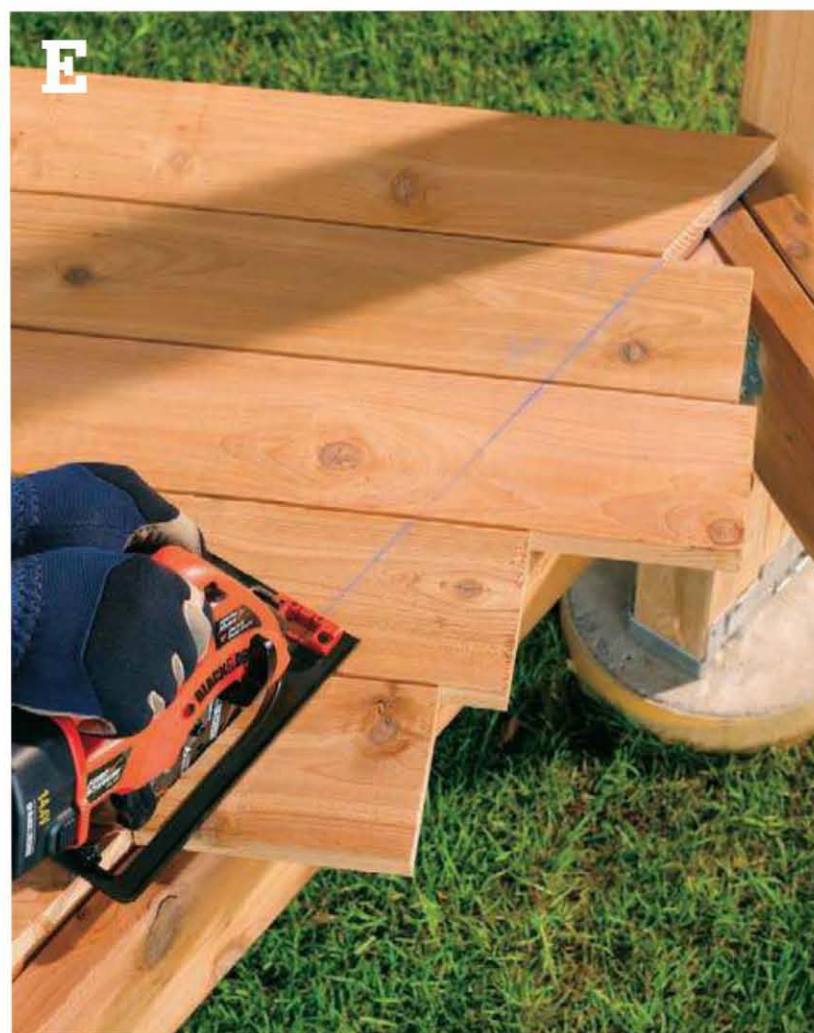
Cut along chalk lines to trim the ends of the decking boards along the floor beams.
