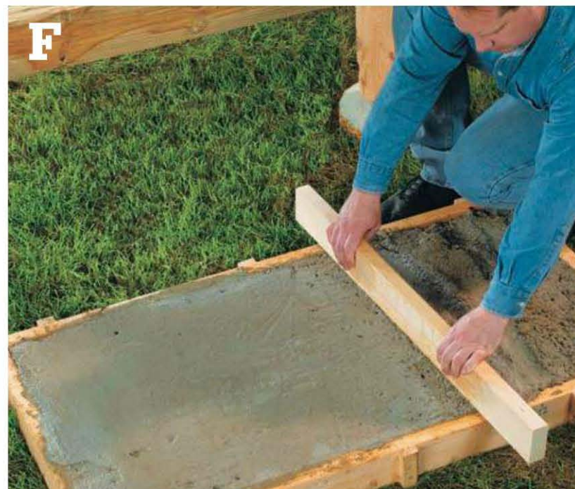
Fill the 2 × 4 form for the stair pad with concrete, then screed the top with a straight piece of 2 × 4.
