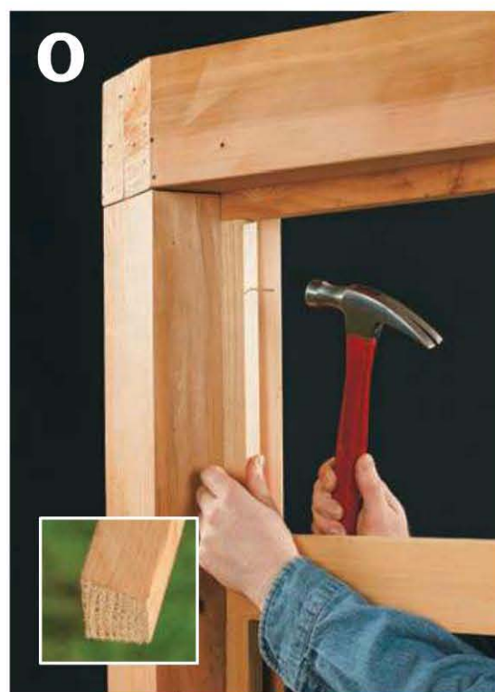
Install the inner stops and rails on the layout lines. The vertical stops are beveled at 22½° (INSET).
