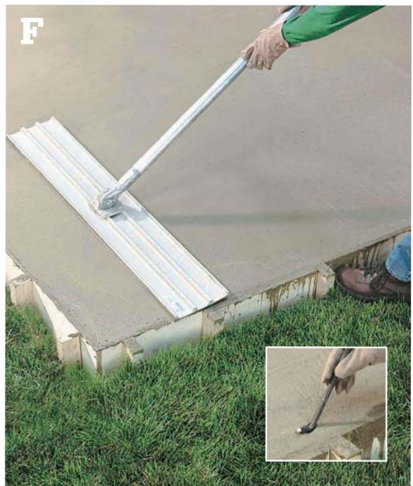
Float the slab with a bull float , then set the J-bolts at the marked locations (INSET).
