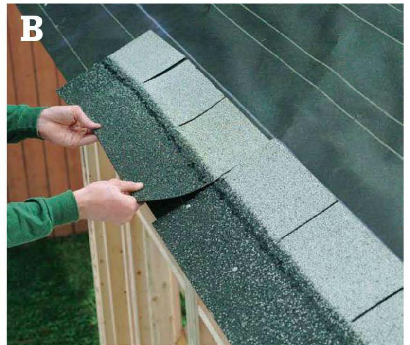
Trim 6" from the end tab to begin the starter row. Position the starter course shingles upside down so the tabs point up.
