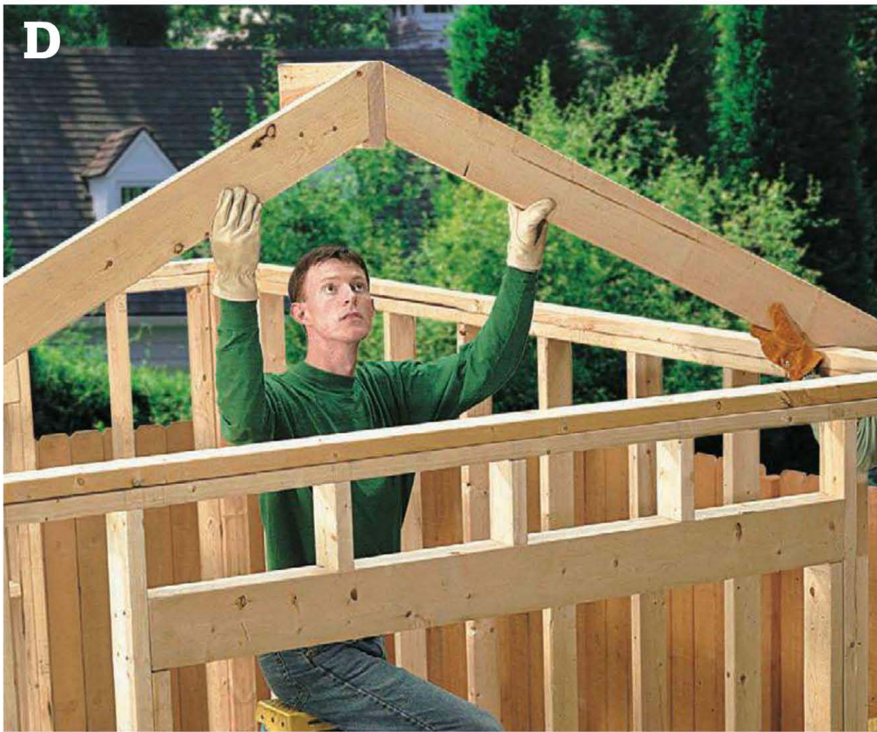
Test-fit the pattern rafters, using a spacer to represent the ridge board or roof hub.
