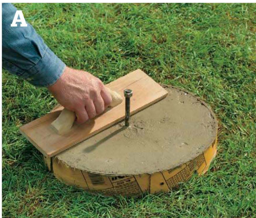
As the concrete sets, finish the tops of the piers using a concrete float.
