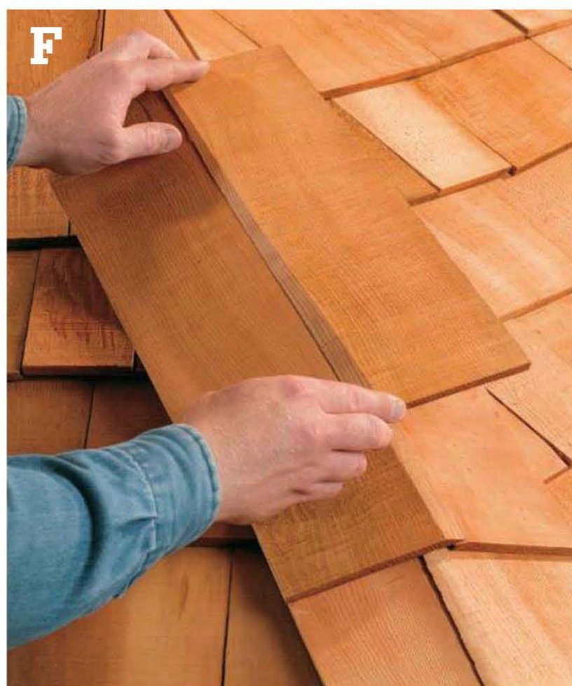
Align pre-made shingle caps over ridges , working from the bottom up.
