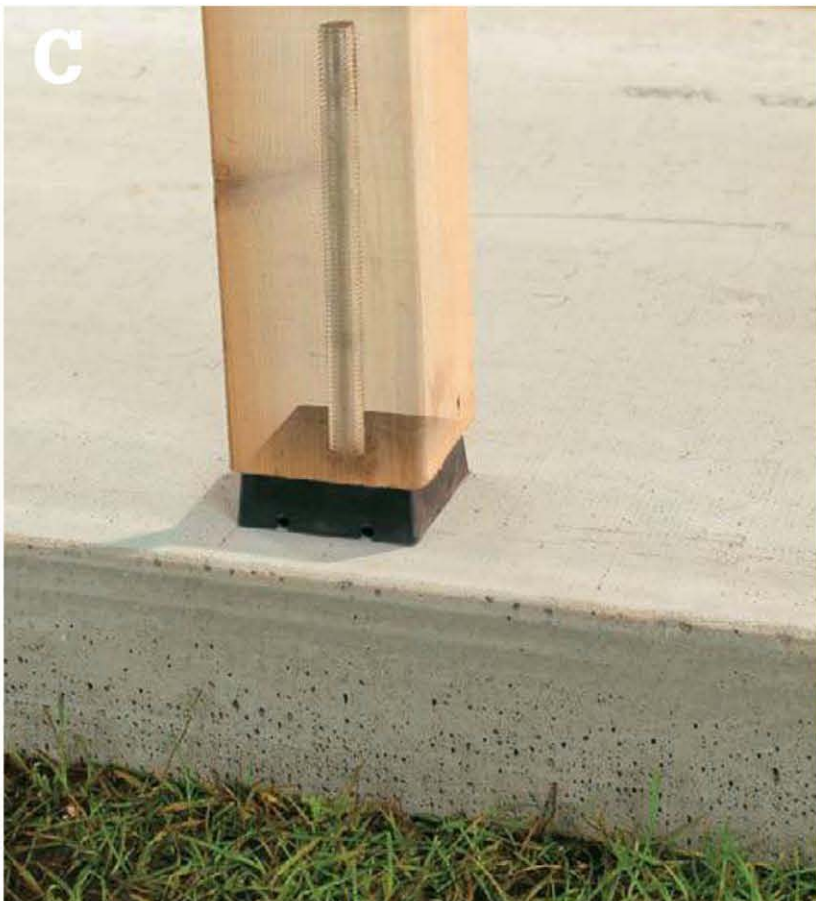
C Set the posts into the slab with anchoring rods —brace them so they are perfectly plumb.
