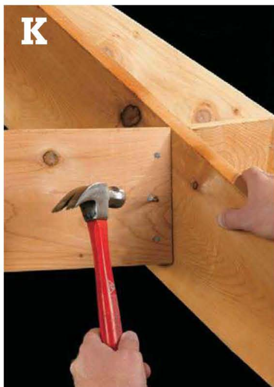
Bevel-cut the ends of the purlins so they meet flush with the rafter faces, and install them between the hip rafters.
