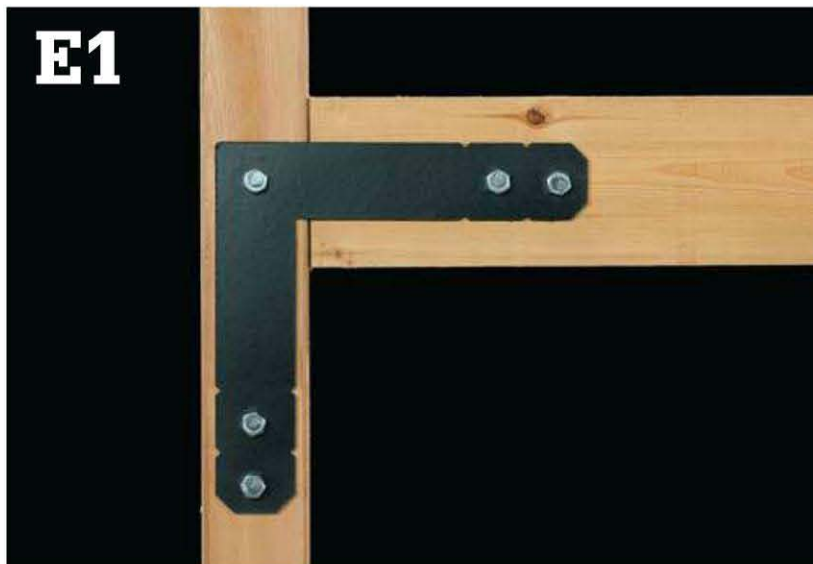
Side wall beam to corner post connection.
