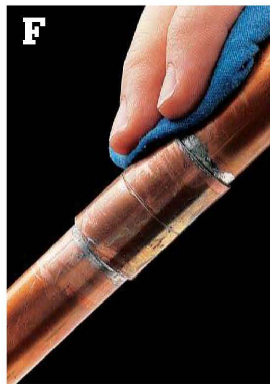
When the joint has cooled , wipe away excess solder with a dry rag. Be careful: The pipes will be hot.
