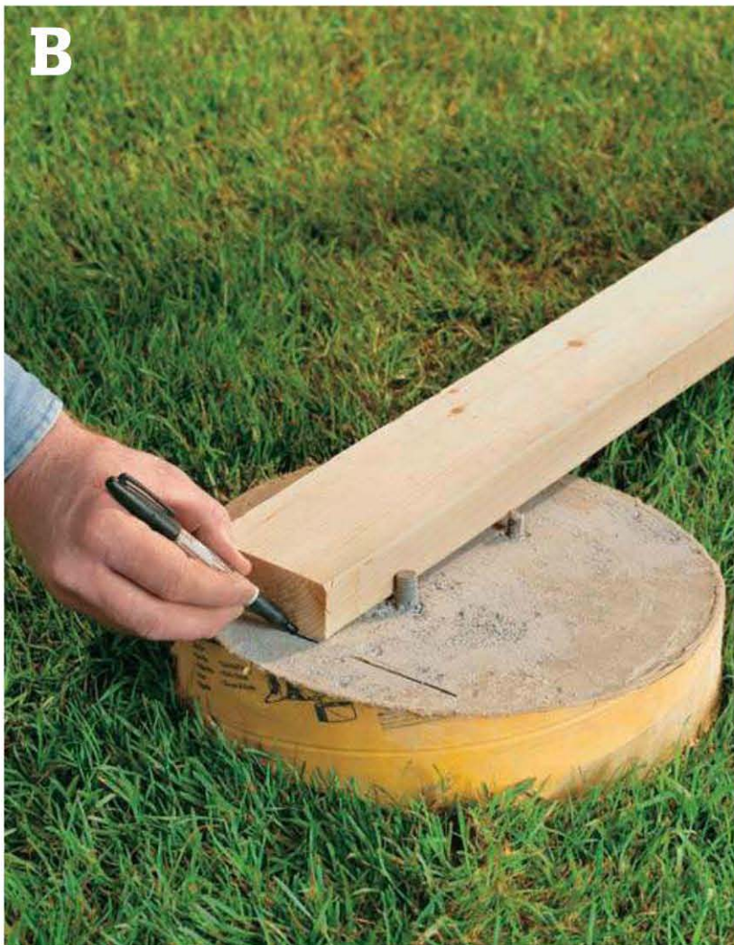
Mark a line across the tops of the piers; this helps ensure all post bases are facing the gazebo's center.
