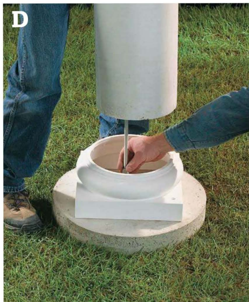
Have one person lift up the column while another tightens the coupler nut to the J-bolt and threaded rod.
