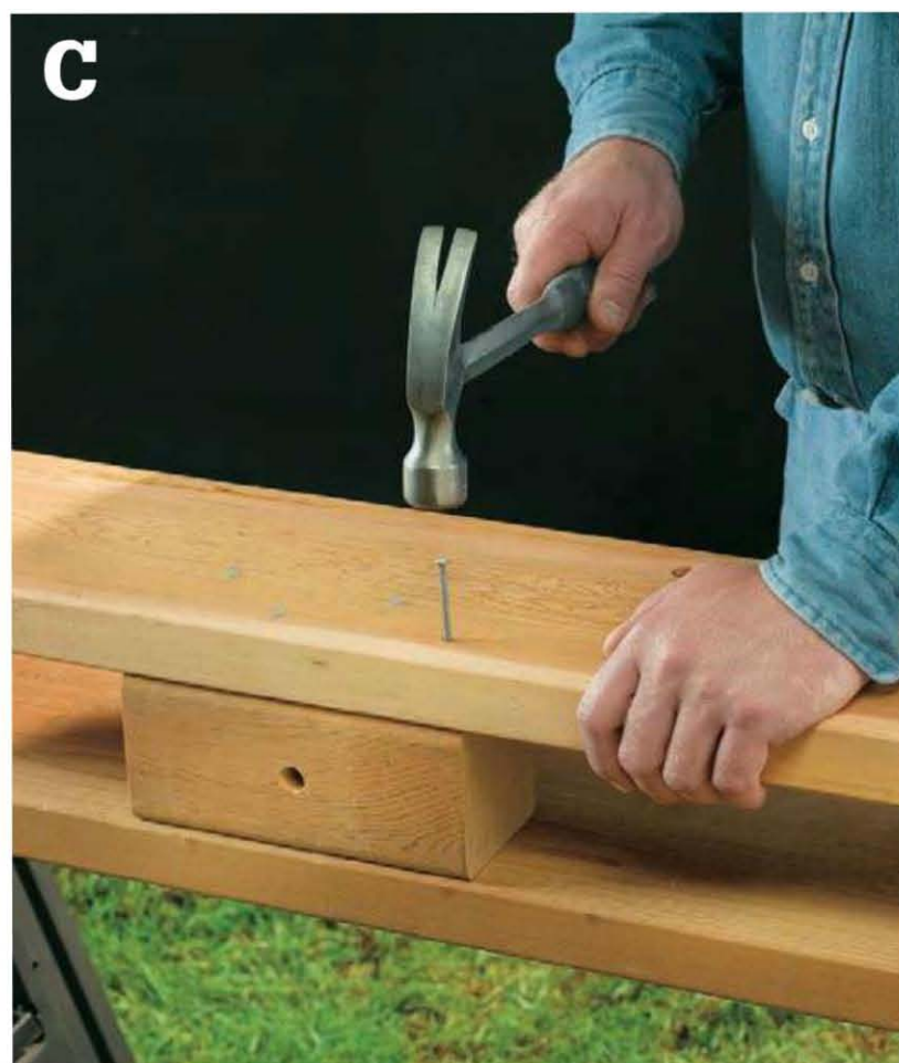
Sandwich the blocks between the main beams, and fasten the assemblies with glue and nails.
