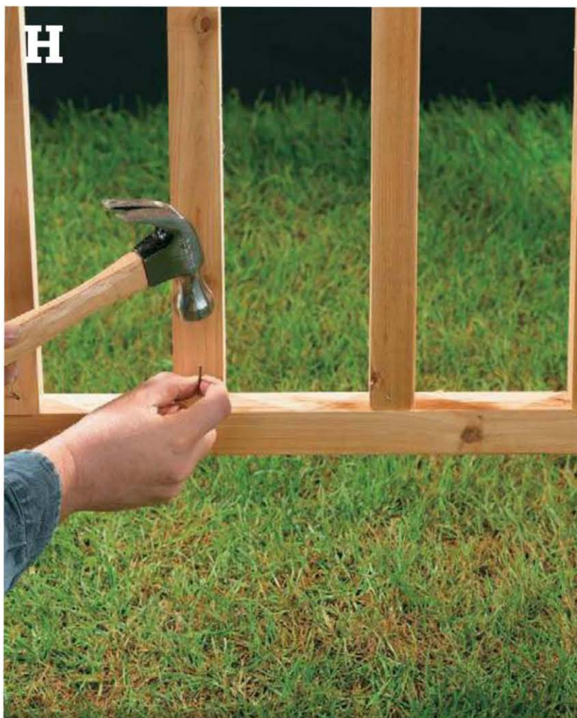
Nail the finish nails into the pickets. To further hide the nail heads, countersink the nails with a nail set.
