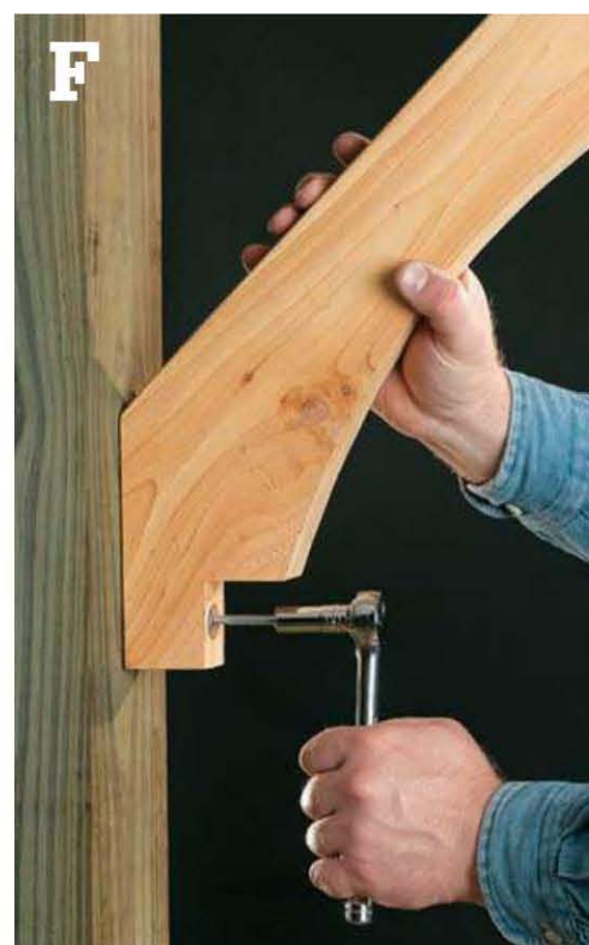
Install the corner brackets so they are centered on the posts and beams.
