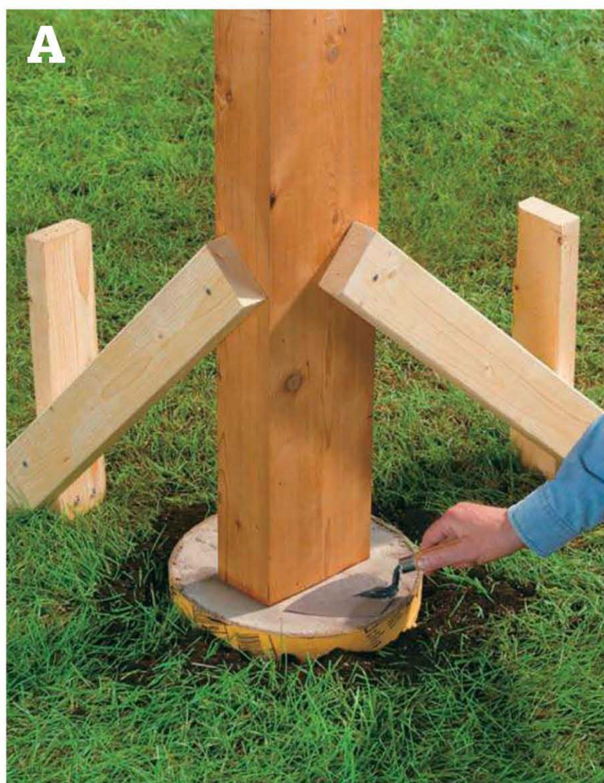
Set the posts in concrete, then cut off the exposed portion of the cardboard tube form.
