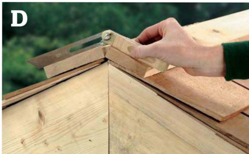
Install the first course of shingles on top of the starter course, offsetting the shingle gaps 1½" between the courses.
