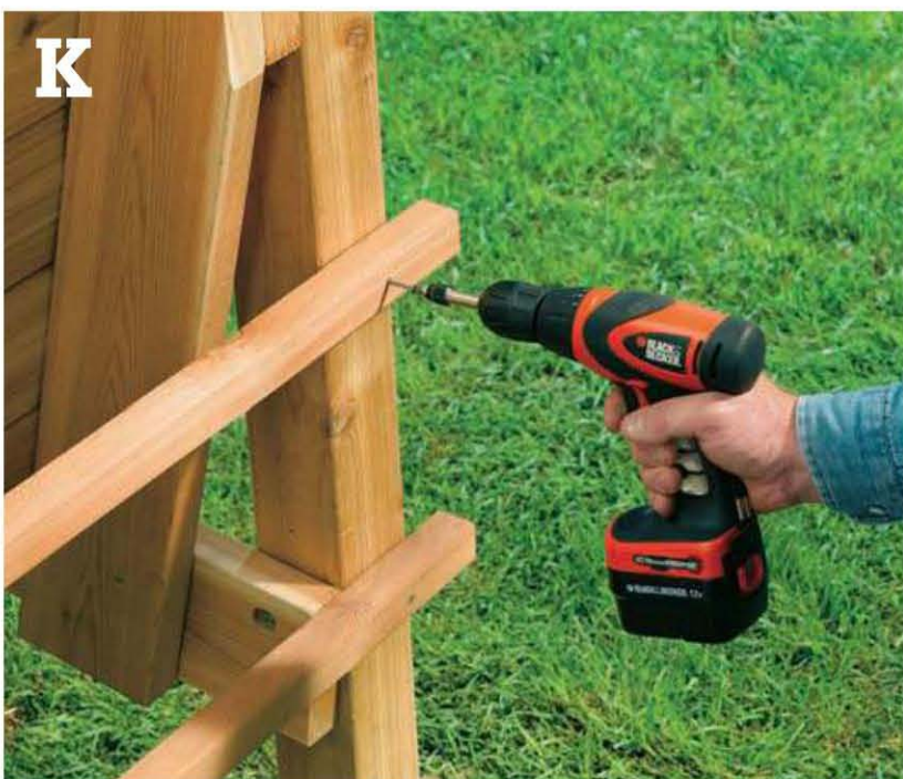
Fasten the back slats to the outer posts with 2½" deck screws.
