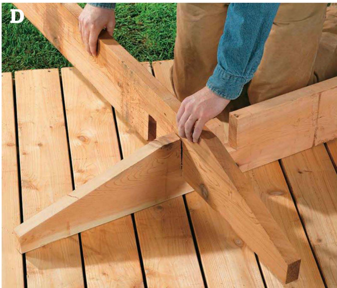
Test-fit the beam joints and make adjustments before installing the beams.
