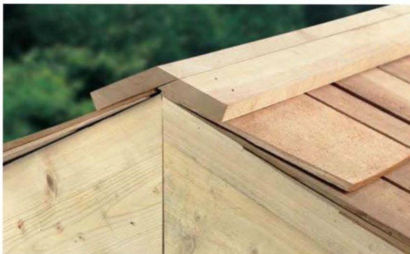
Use a T-bevel and scrap boards to find the ridge angles (above), then cut the 1 × 4 and 1 × 6 for the ridge cap.
