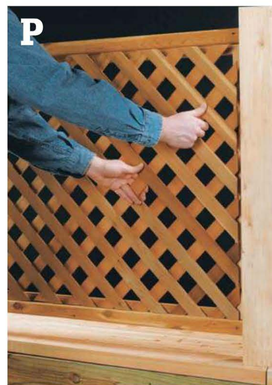
Set the lattice panels against the inner stops and rails, and fasten them with 3d galvanized finish nails.
