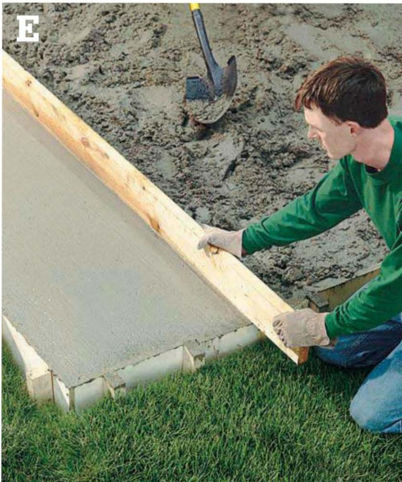
Screed the concrete after filling the form, using two people to screed, while a third fills low spots with a shovel.
