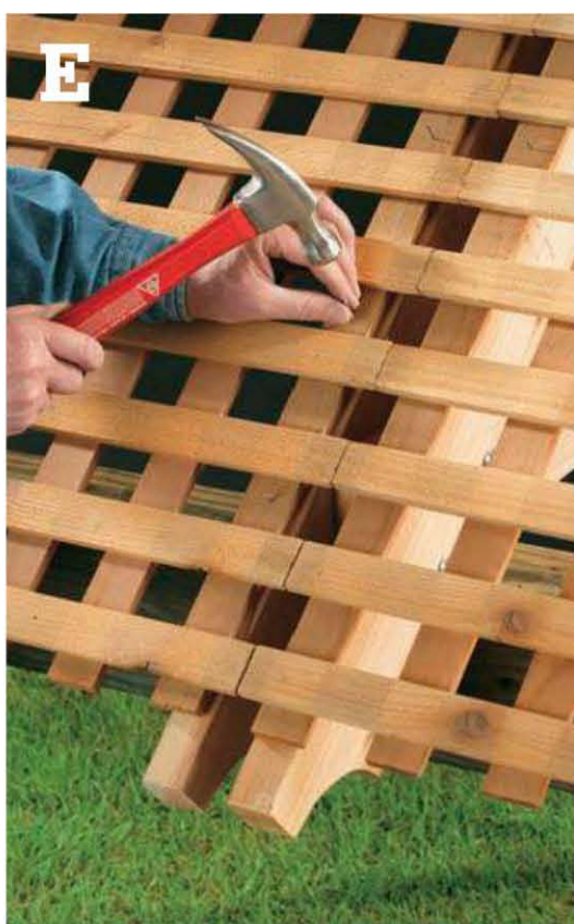
Install the roof panels so the seams fall over the center truss and the ridge boards.
